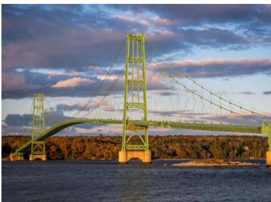
Figure 1.12: Deer Isle Bridge
