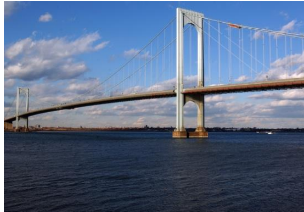
Figure 1.11: Bronx-Whitestone Bridge, New York
