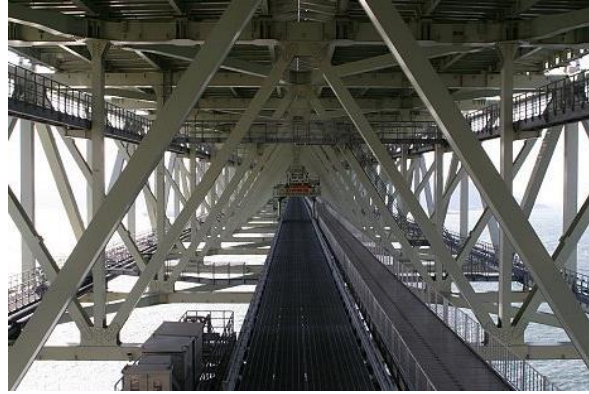
Figure 1.24: Akaishi-Kaikyo stiffening truss
