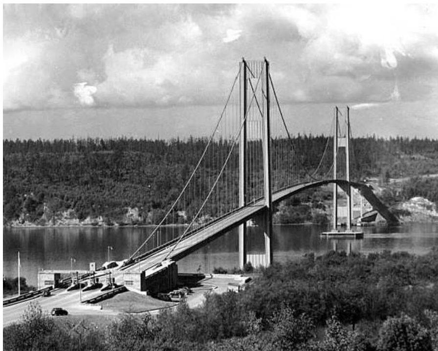
Figure 1.16: Original Tacoma Narrows Bridge
