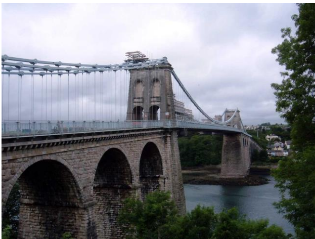
Figure 1.3: Telford's Menai Straits Bridge, Wales
