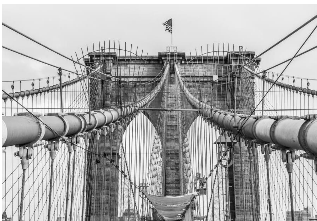
Figure 1.6: Brooklyn Bridge main cables and stays
