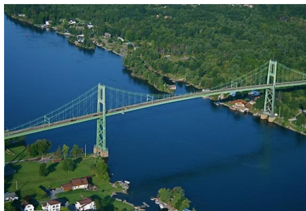
Figure 1.13: Thousand Island Bridge
