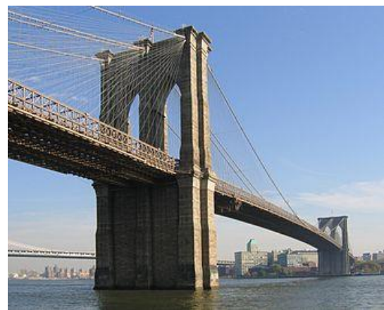
Figure 1.7: Brooklyn Bridge, New York
