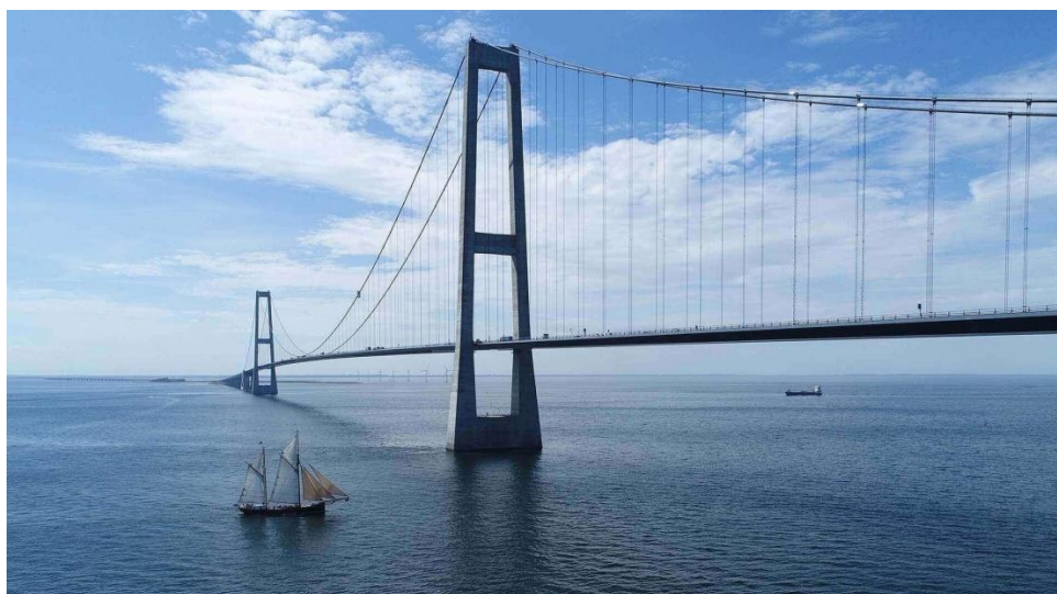
Figure 1.22: The Great Belt Bridge
