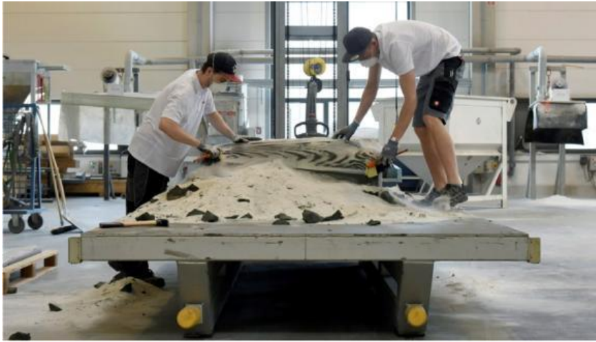
Figure 18 – Post-processing of the 3D printed formwork parts. Unconsolidated sand particles are being removed from the print bed
