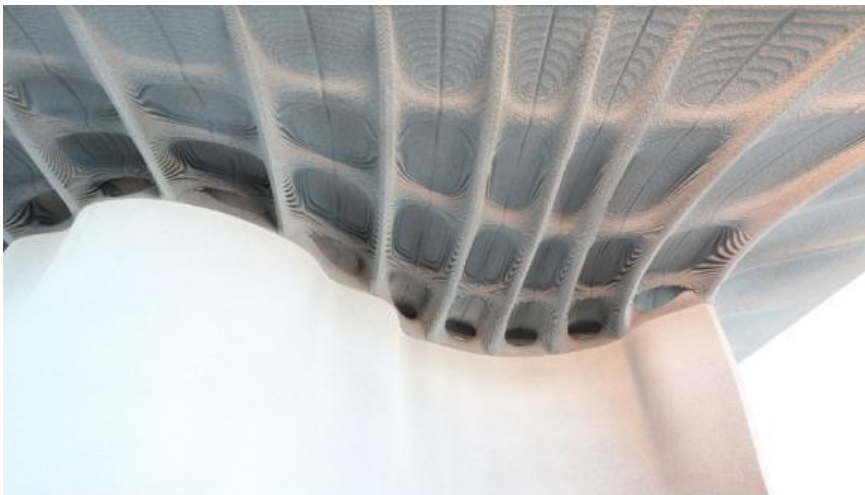
Figure 19 – complex shape of the ceiling obtained with 3D printing
