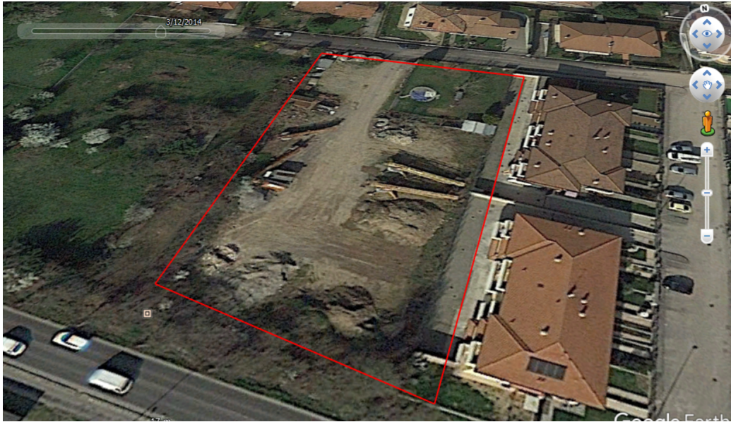
Figure 5.1: Construction leftovers in urban area
