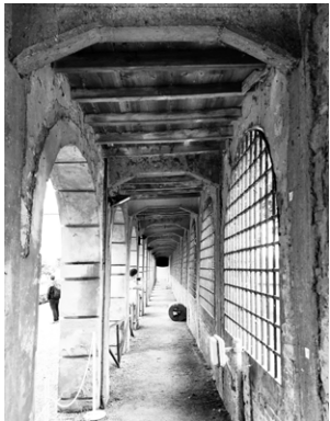
Figure 52: Existing Situation of Restored portico
