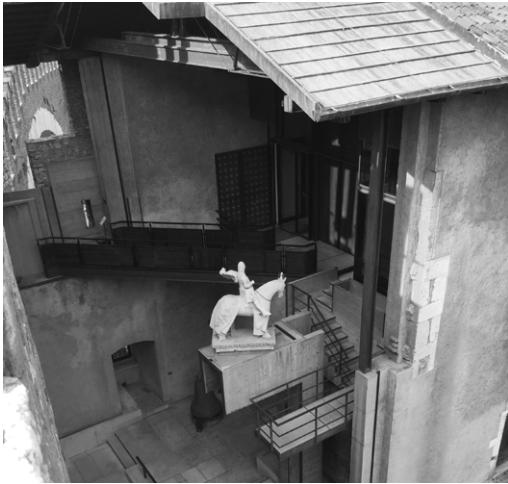
Figure 44: View of the connection part between the two volumes of Castelvecchio
