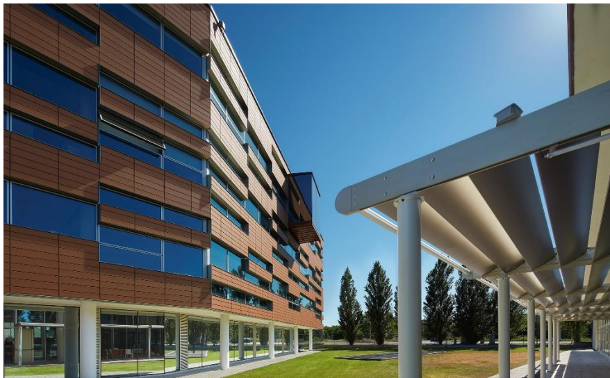
Figure 48: Shows the sunshades that prevent sun rays from the glassed facades (Source: [203]).
