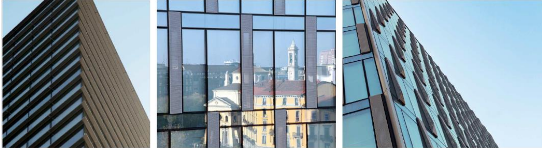
Figure 43: Sunshades on Varesine Office Building (Source: [202])
