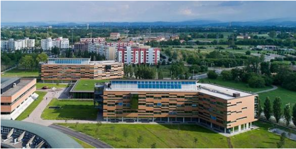
Figure 49: Shows the Photovoltaics Panels on the roof (Source: [203]).
