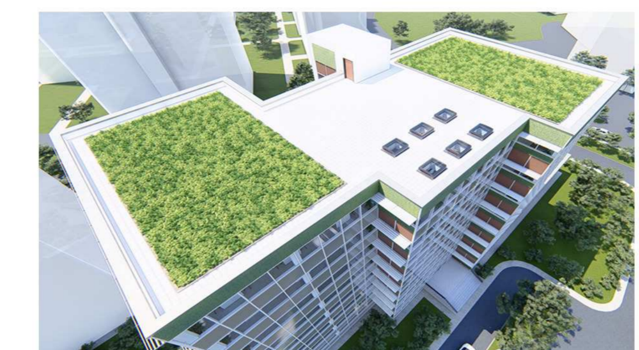
The Green Roof and the Skylight on the Roof of the Building
