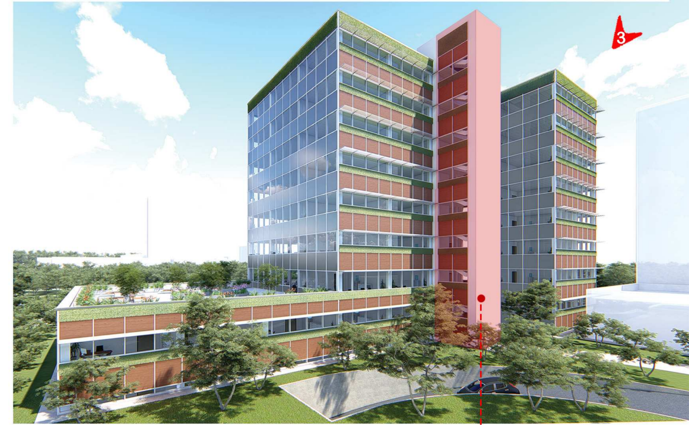
The Intervention of Renovate a Service Stairs to work as Solar Chimney in the South West Facade
