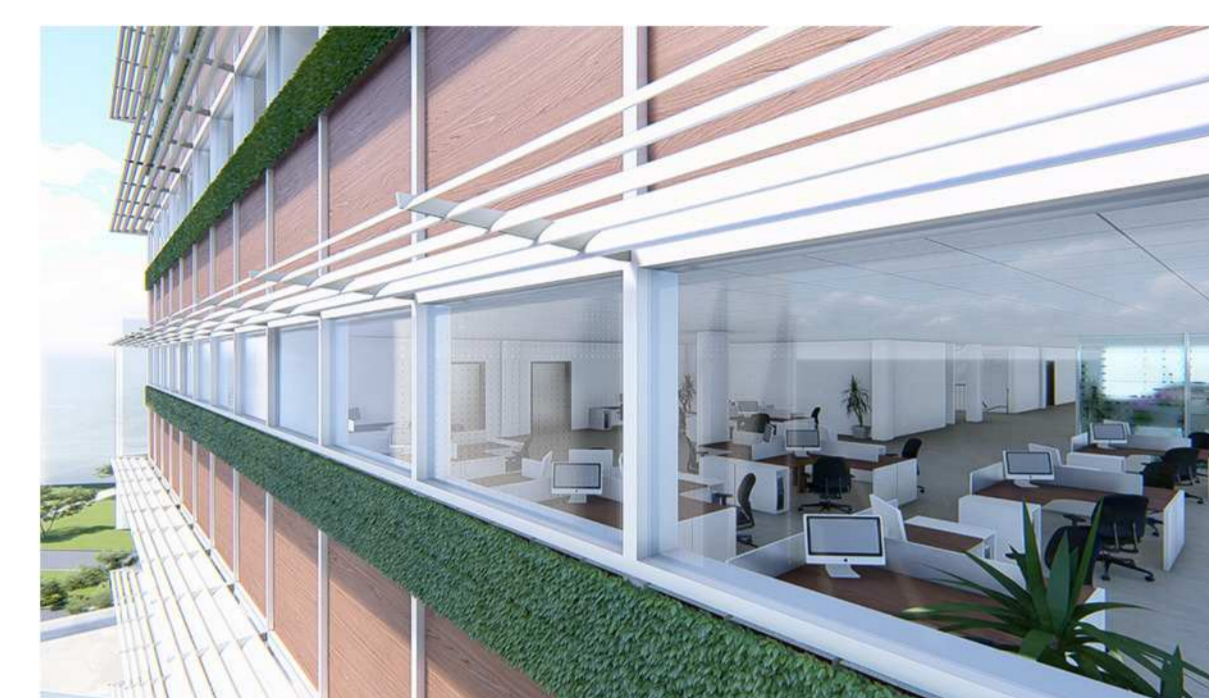
The Horizontal Sunshades in the (South East & South West) Facades
