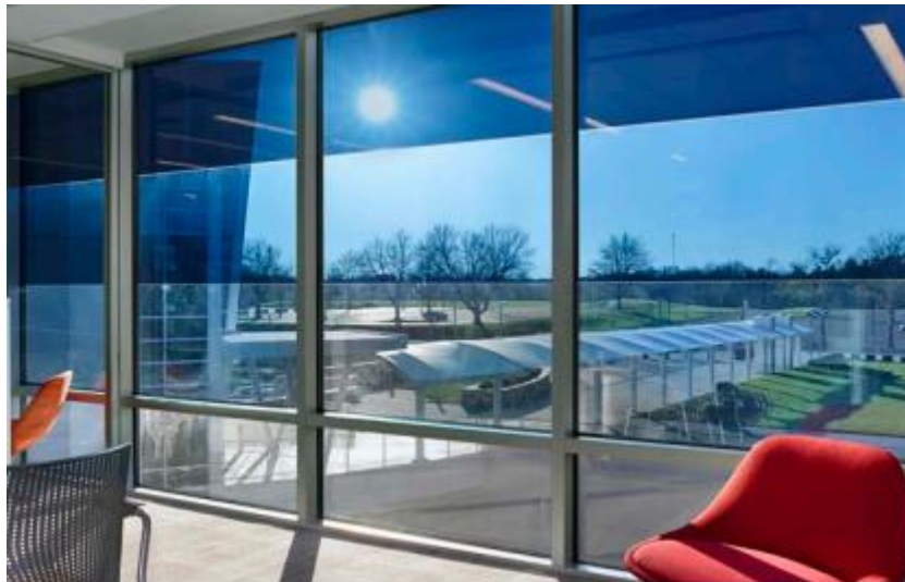
Figure 1-3 Electrochromic dynamic glazing Sage LightZone ® (22)
