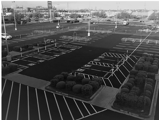
conventional: impervious asphalt pavement surface parking area
