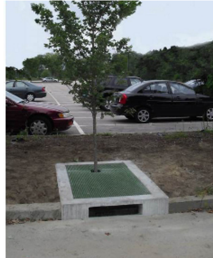
Tree filters can collect stormwater through an attached a curb inlet in Boston..
