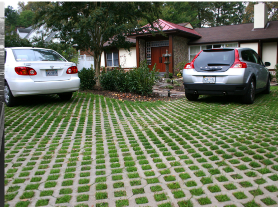
LID: pervious surface pavement parking area
