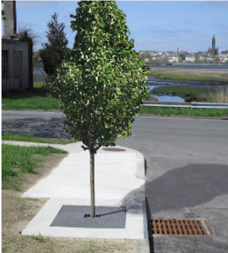
Tree filters can collect stormwater through an attached a curb inlet in Boston..
