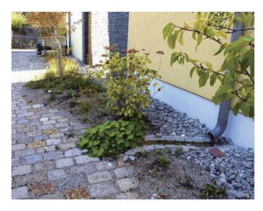
Stone swale: Arranged under the rainwater pipe. A considerable part of the vegetation in the plantation is also planted and maintained by the residents themselves. This will trap some of the rainwater, and the excess rainwater will spill directly into the grass or water storage facilities.
