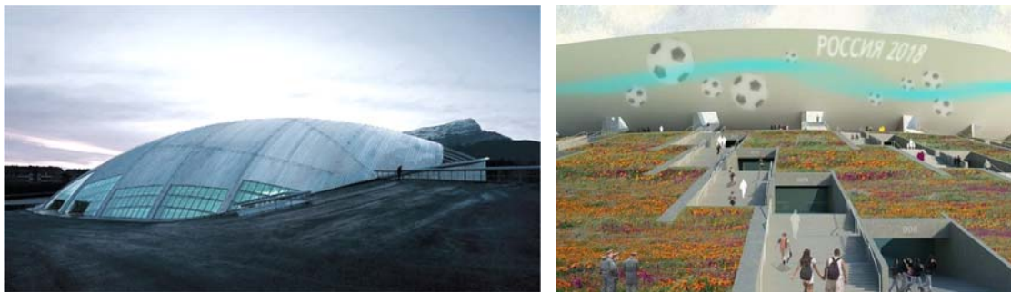
Fig. 4-1-42: Interface Between the Roof of City of Jaca Hockey Arena and the Ground (Coll-Barreu Arquitectos)
