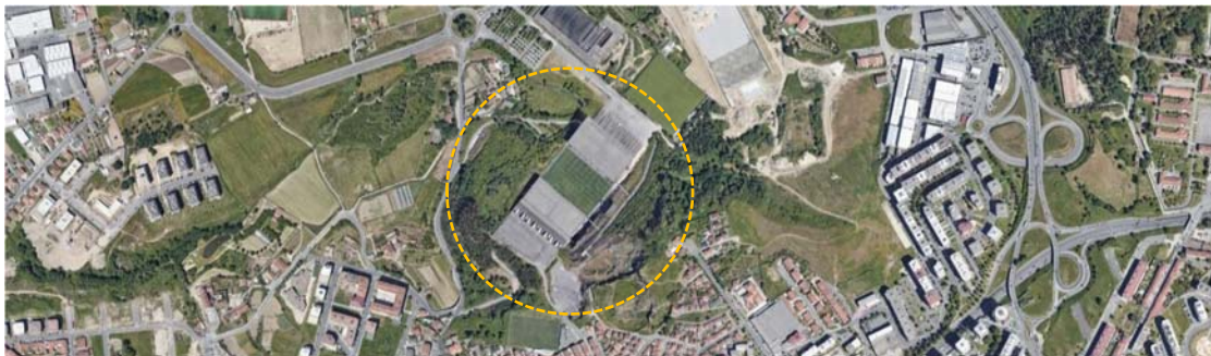
Fig. 3-1-77: The Environment Map of Estádio Municipal de Braga (Eduardo Souto de Moura)
