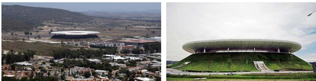
Fig. 3-1-92 & 3-1-93: Distant View and Street View Images of the Stadium
