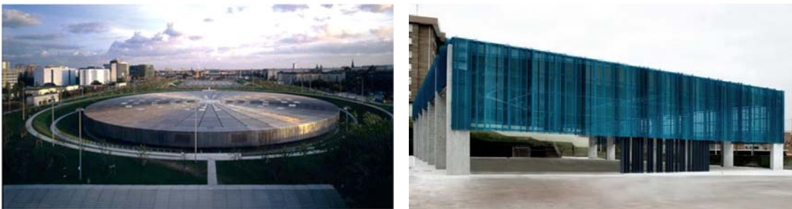
Fig. 4-1-30: Metal Roof of Berlin Olympic Swimming Pool (Dominique Perrault)
