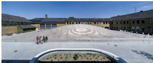
Fig. 3-1-27: Image Viewing from the Yard
