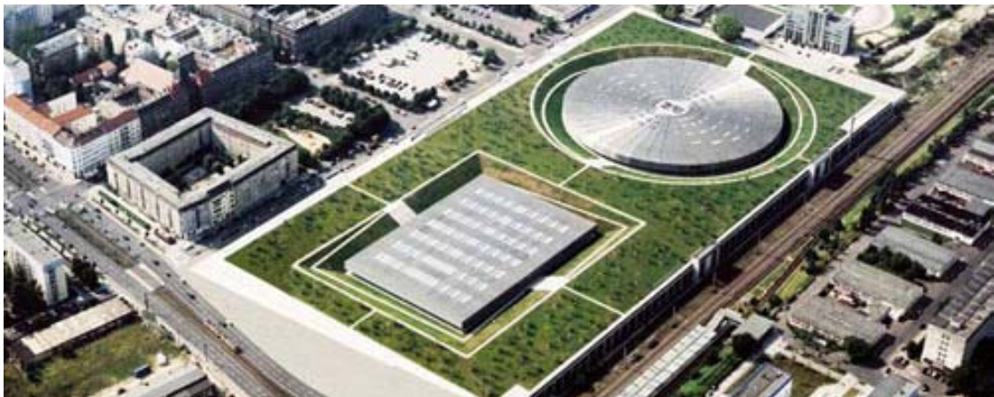
Fig. 3-2-2: Bird View Image of the Site and Buildings
