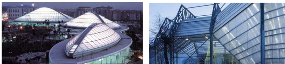
Fig. 4-1-32: Roof Interface of Guangzhou New Stadium (Paul Andreu)
