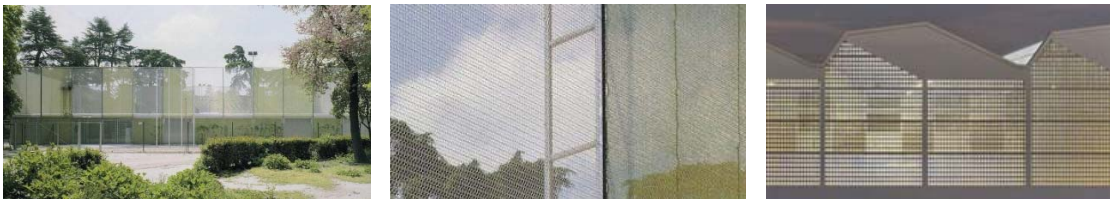
Fig. 4-1-38 & 4-1-39: Facade of Gymnastics Pavilion
