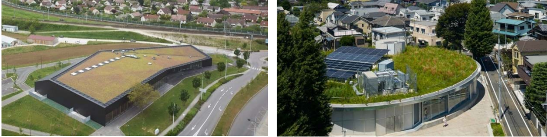
Fig. 4-1-26: Roof Interface of Longvic Sports Center (Dietrich | Untertrifaller Architekten)
