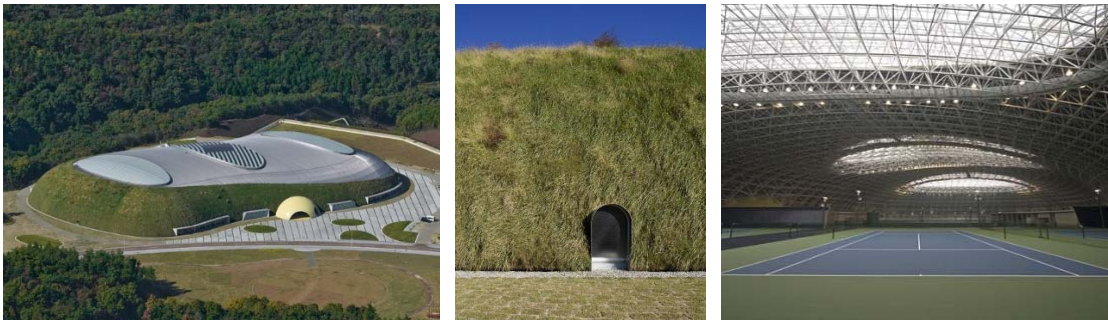
Fig. 3-1-17 & 3-1-18 & 3-1-19: Bird View, Plant Surface and Internal Space Images of Slowtecture M (Shuhei Endo) Description: The physical environment inside is adjusted mainly because of the surface design. Soil covering is common in landform buildings since it is a sustainable approach and integrate the building into the natural environment. Source: www.archdaily.com/6853/slowtecture-m-shuhei-endo/
