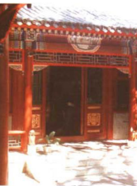
View of north room from west room
