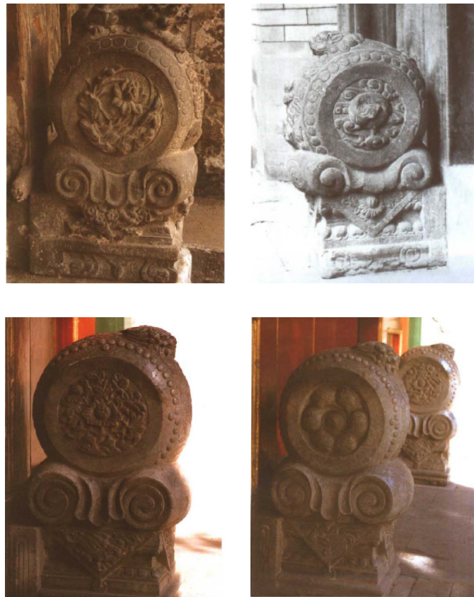
Examples of drum-shaped bearing stone
