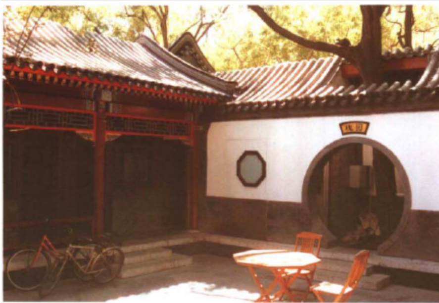
View of east room from northwest corner
