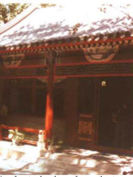
View of west and north room from southeast corner
