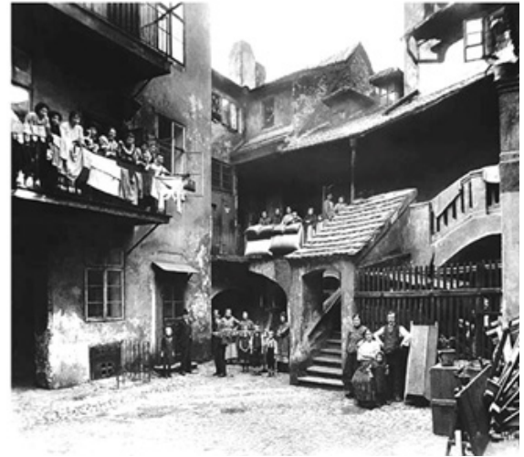
2.11 . The demolition of houses near the Church of the Holy Spirit and the Spanish Synagogue.
