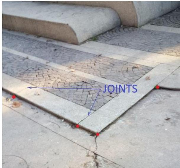
*Figure 4.3: Joints between stones and several example points measured with Leica GRX1200*
