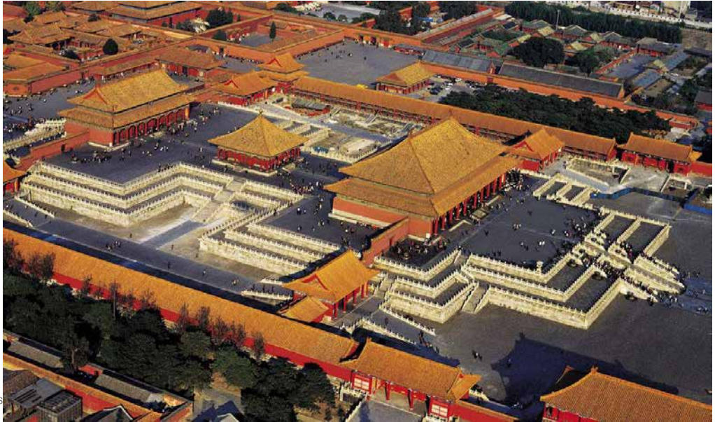
Fig. 4.12 Aerial View of Three Great Halls Source: pic.baidu.com
