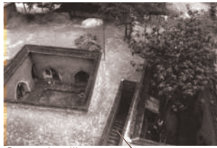
Cave dwelling Gansu Province, Shanxi Province, Shanxi Province, Henan Province, Hebei Province, Ningxia Province
