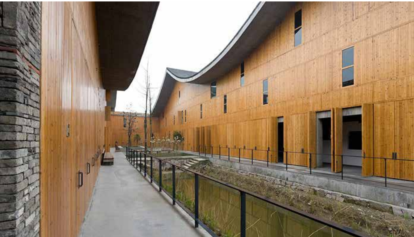
Fig. 1.20 New Academy of Art in Hangzhou / Wang Shu, Amateur Architecture Studio Source: Sharon Lam. Focus: Wang Wei. https://www. archdaily.cn/ cn/801319/jiao- dian-wang-shu
