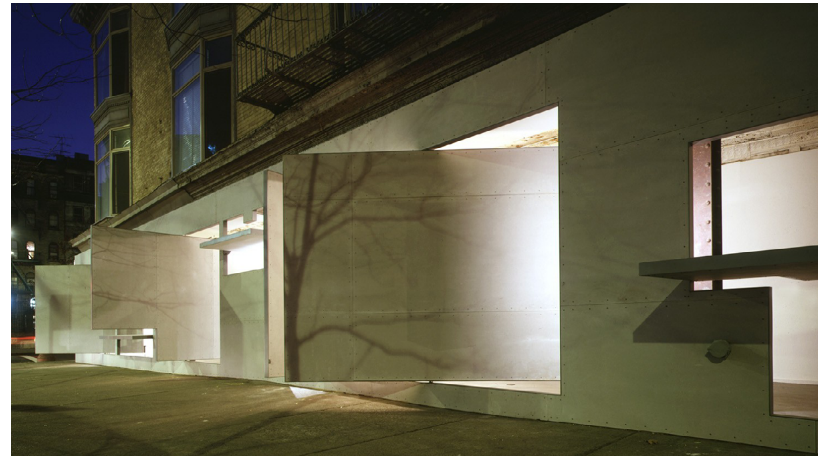
Fig.17 Facciata mobile dello Storefront for Art and Architecture dell'architetto americano Steven Holl Mobile facade of the Storefront for Art and Architecture by the American architect Steven Holl
