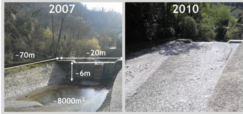
Figure 1.2: Retention Basin on Caldane River, topped up in three years
