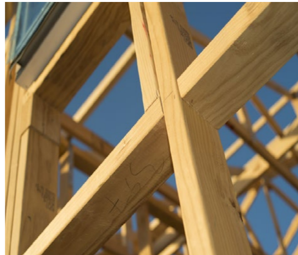
Figure 1.1 - The timber frame of a building
