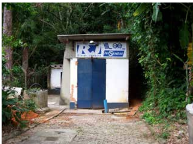
Figure 3.3.4 Water lift station EE1. Source: Planave S.A.
