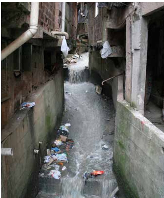
Figure 1.4.5 Most of the waste and sewage from the favela runs through open sewers like this one in Rocinha. Source : ROCINHA.ORG "O Portal da Rocinha Real".
