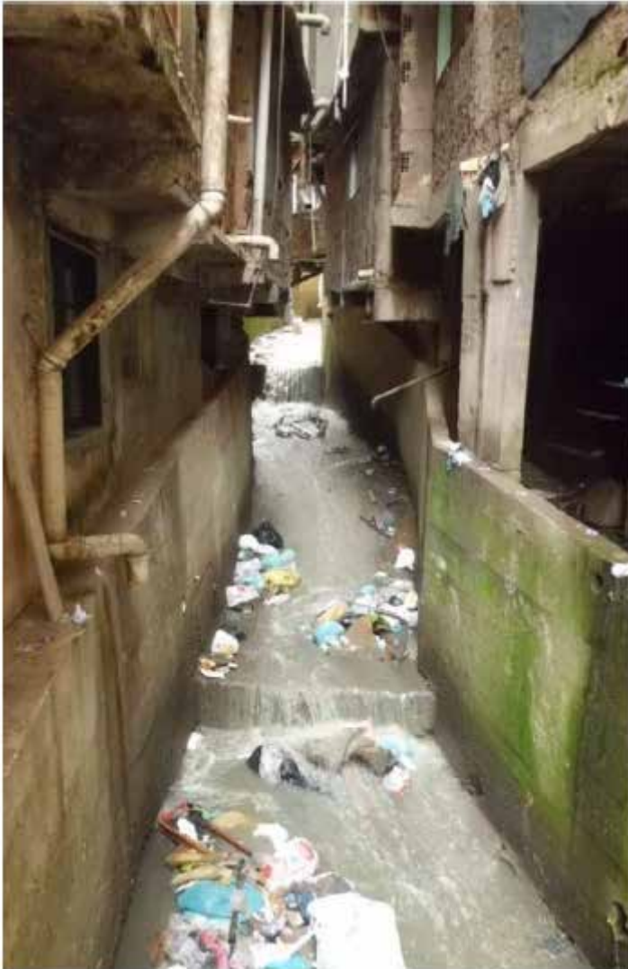
Figure 3.3.20 Discharge of sewage directly into a talvegue. Source: CONEN, 2012
