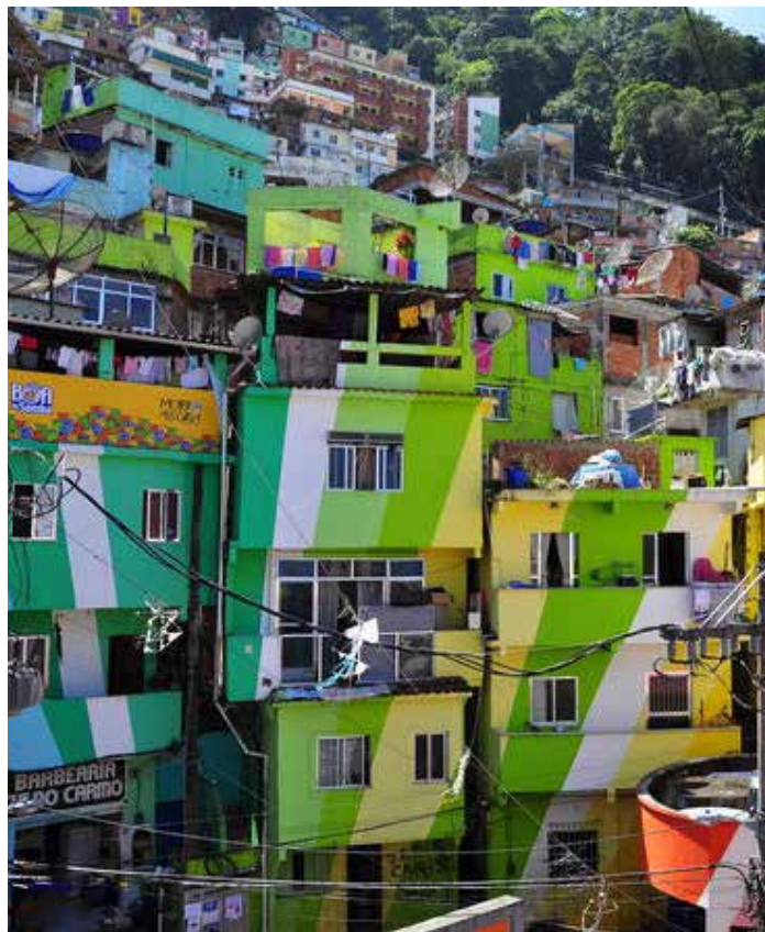
Figure 5.1.20 Façades refurbishment in the Santa Marta favela, RJ. Source: www.wiztours.com
