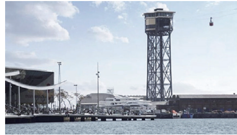
4| Alta Mar Tower
