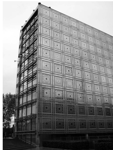
Figure 3.16; Arab World Institute was designed by Jean Nouvel with a kinetic facade system
