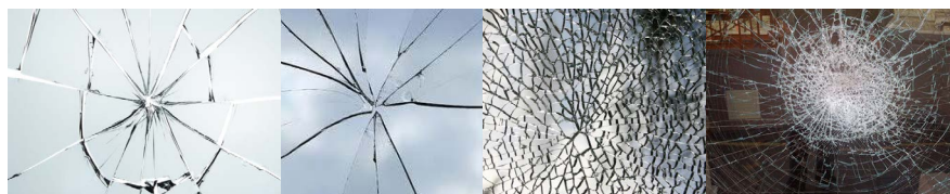
a) Annealed glass b) Heat-strength glass c) Tempered glass d) Laminated glass
