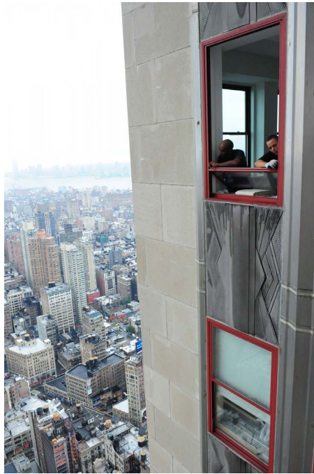
Figure 3.54; Retrofitting process on the site
