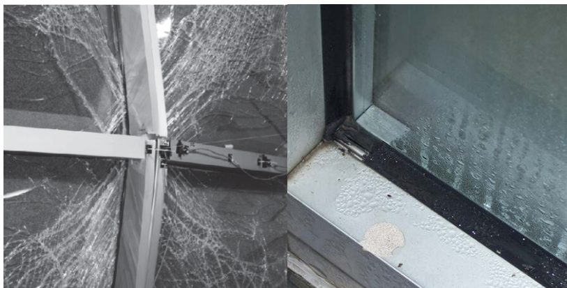
Figure 3.41; Various framing failures of the curtain wall
