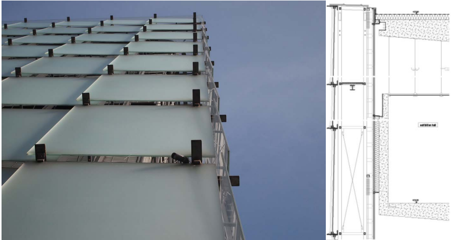
Figure 3.18; The Kunsthaus was designed with translucent panels on the facade
