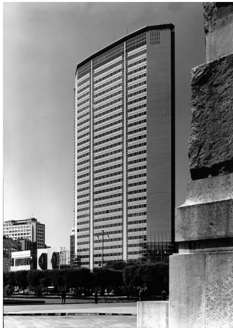
Figure 2.2; Pirelli Tower, Milan
