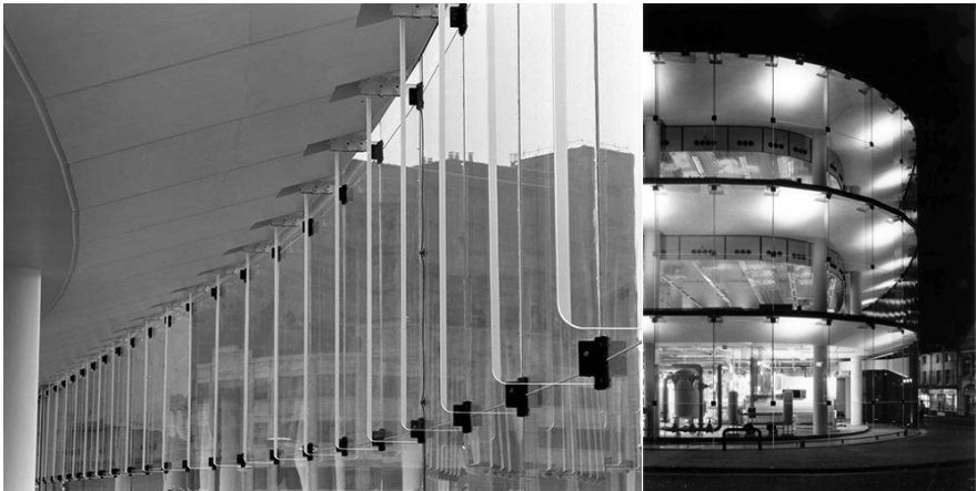
Figure 3.14; Facade of the Willis Faber and Dumas Headquarters was designed with structural glazing system
