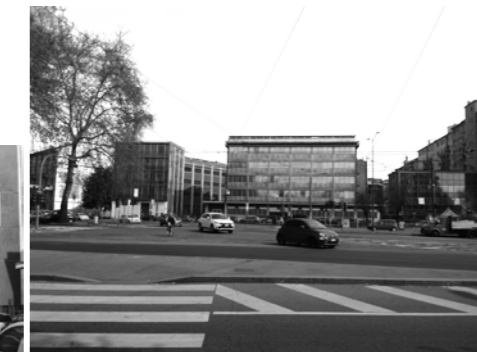
Abandoned Office Complex
