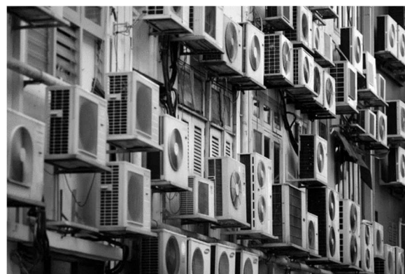
Figure 11, a typical building relying on the air condition
