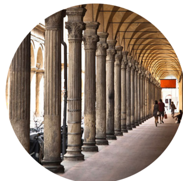
Continuous Porch, Bologna
