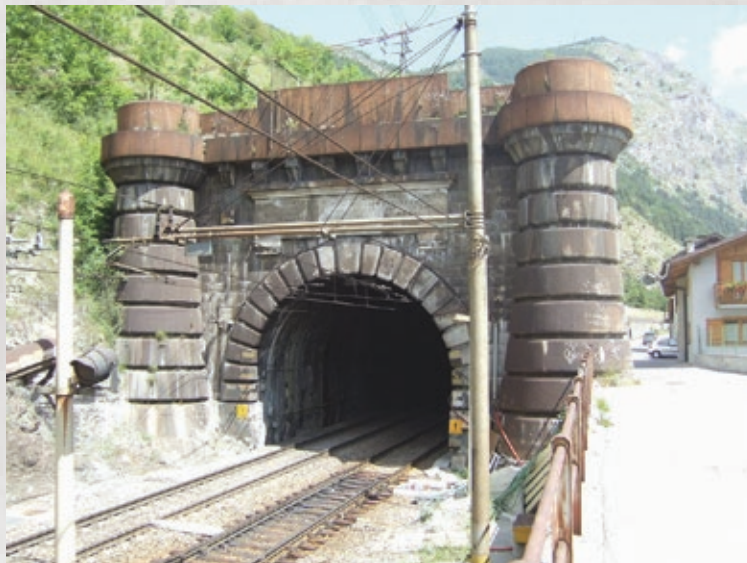
1.6 Fréjus Rail Tunnel
