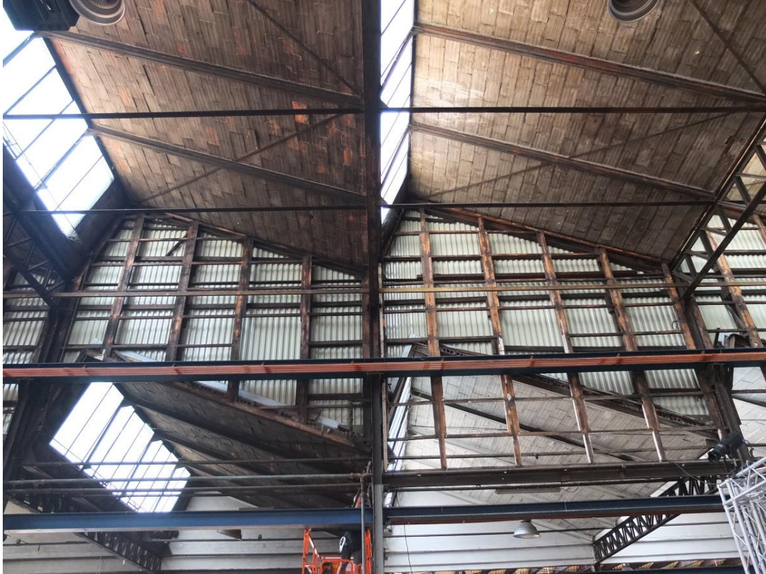
Figure 95. The layer of inclined roof in the building
