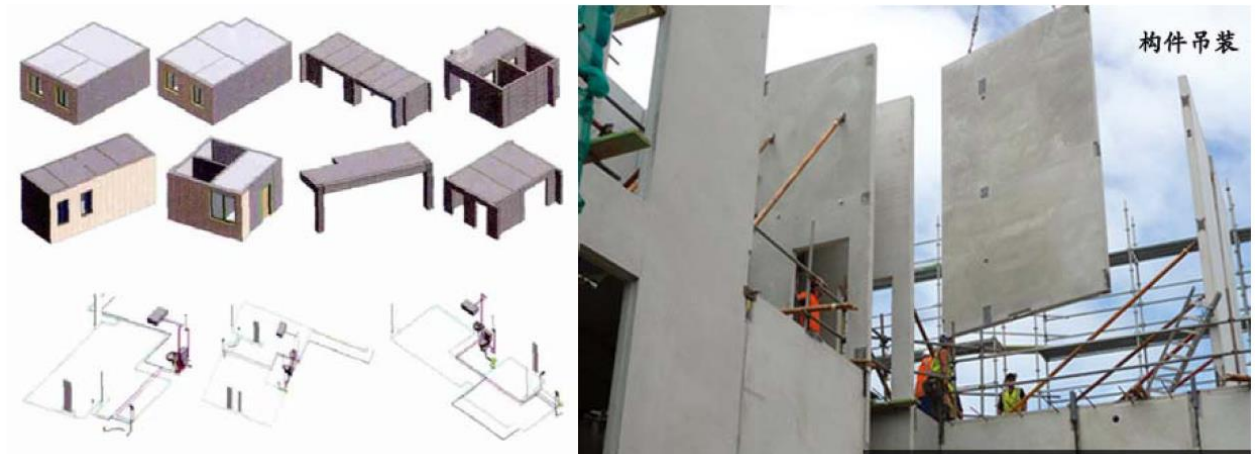
Figure 48. Various units at different scales and building components in construction site (source: Zhanga et al., 2016)
