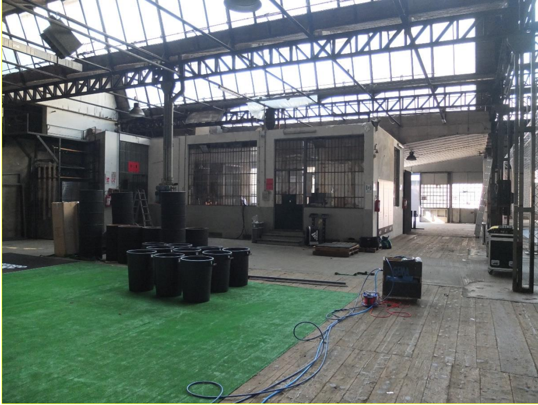
Figure 93. Floor type 2 in the building
