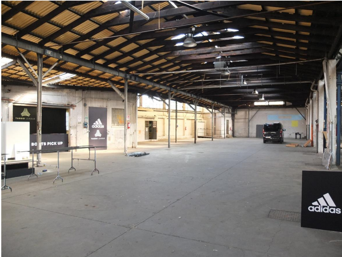
Figure 91. Floor type 1 in the building
