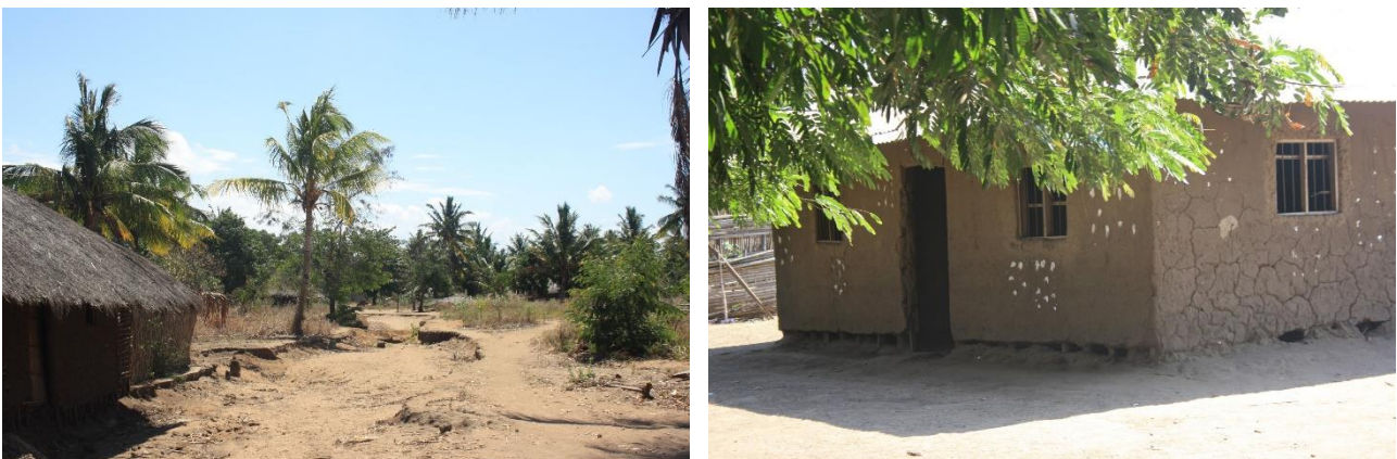
Figure 10 Evidences of the passage of Cyclone Kenneth in the village of Nanjua (left) and Namuapala (right)
