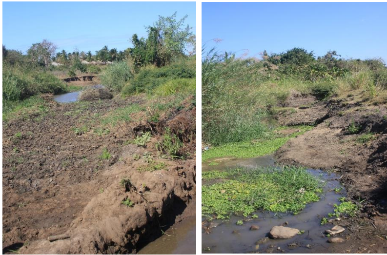
Figure 13 Photos from field survey depicting a branch in fair condition
