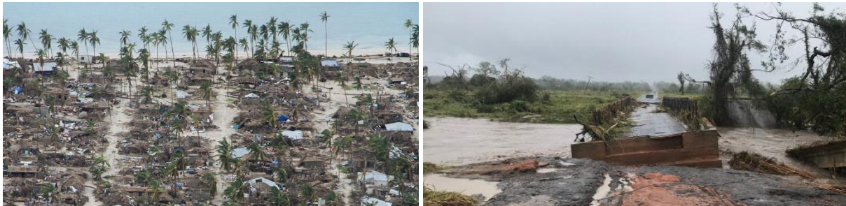
Figure 23 Effect of the Cyclone Kenneth on a village in Cabo Delgado up, damaged bridge down
