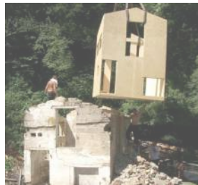
Dovecote Studio, Haworth Tompkins 2010 - Suffolk, UK
