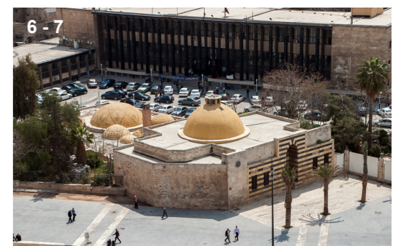
6-7 Hammam Yalbougha al-Nasiri - XIV century overall satellite damage assessment: SEVERE
