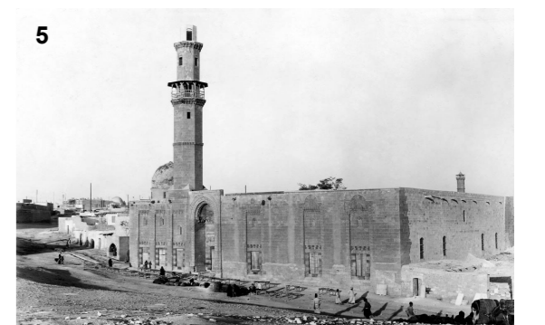
5 Al-Utrush Mosque - 1565 overall satellite damage assessment: MODERATE
