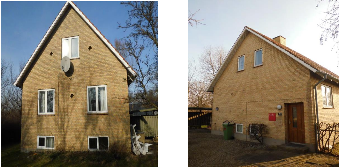
Fig. 2.1: front view (left) and rear view (right) of Flexhouse_03
