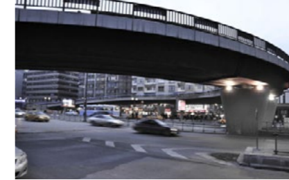
Highway bridge for U-turn in Sıhhiye
