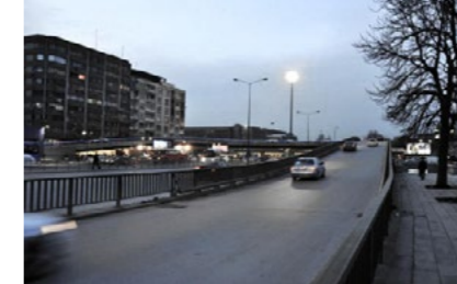
Highway bridge for U-turn in Sıhhiye
