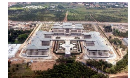
Construction of governmental facility, 2015.
