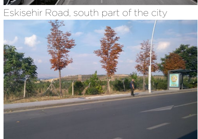
Sidewalk in Eskişehir Road, behind is AOC
