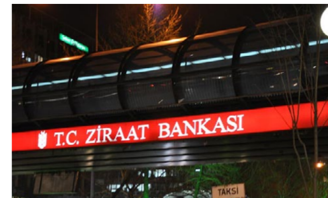
Overpass in Kizilay
