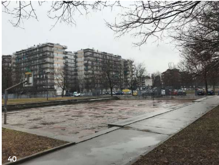
Figure 40. An example of the numerous open public spaces in the area of Satellite. Source: author
