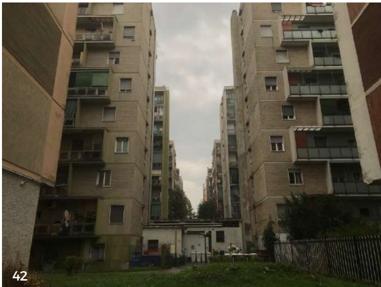
Figure 42. Innards of the critical blocks of Satellite. Source: author
