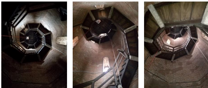
Fig. 8.2. Bell-tower of the church of San Gottardo in Corte: internal view of the bell-tower, the circular wooden staircase and the only wooden floor of the building.
