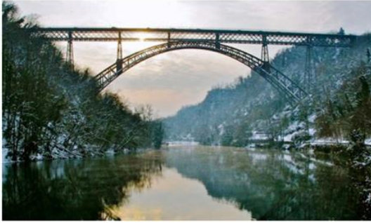
Fig. 6.10. View of the San Michele Arch Bridge
