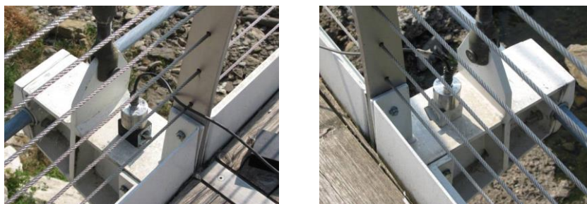
Fig. 4.12. Typical mounting of the accelerometers on site.
