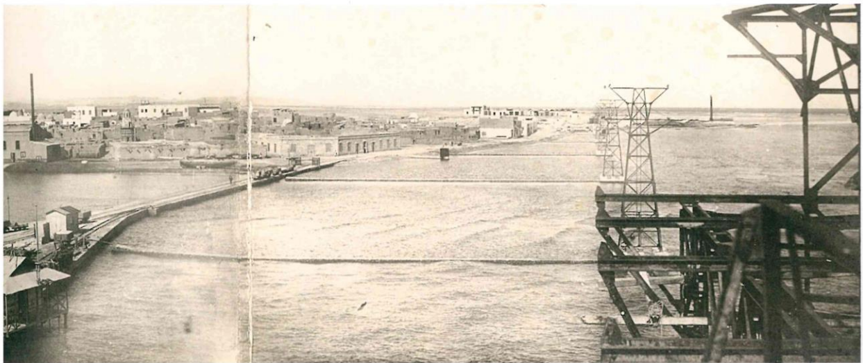
Figure (31): A view of Quseir’s mining town. Source: Antonella Cabassi, Kosseir, A Phosphate Shipping Town: Building Beyond the Mediterranean, Studying the Archives of European Businesses (1860-1970) .
