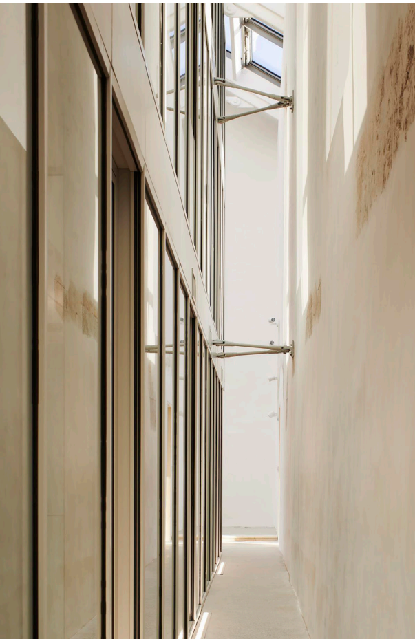
FIGURE 29 _ The St. Luke's Church, Dublin, Ireland: Alterations Do Not Touch Existing Historic Structures.
