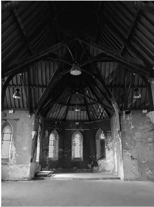
FIGURE 51 _ The Church of Ireland, Grangegorman, Dublin, Ireland: Today.
