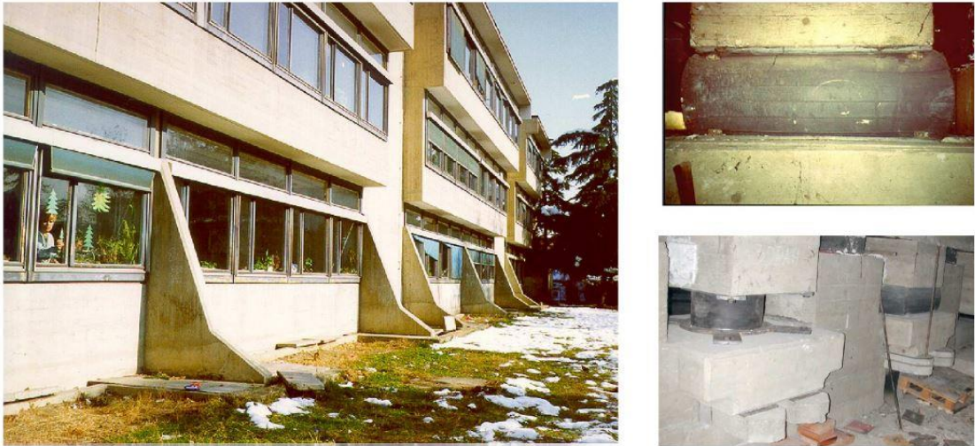
Fig. 1. 5. School building in Skopje isolated with blocks of low-damping natural rubber without reinforcements, causing the rubbers swell sideways [10]. In the last Fig., an isolator was replaced by a new high-damping rubber, next to the original one
