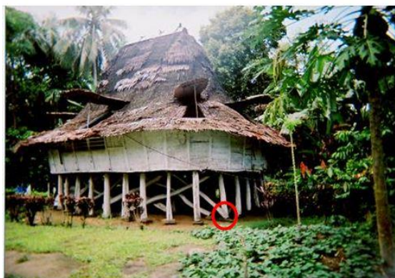
Fig. 1. 3. Sliding foundation of a timber traditional house in Nias Island, Indonesia [8].
