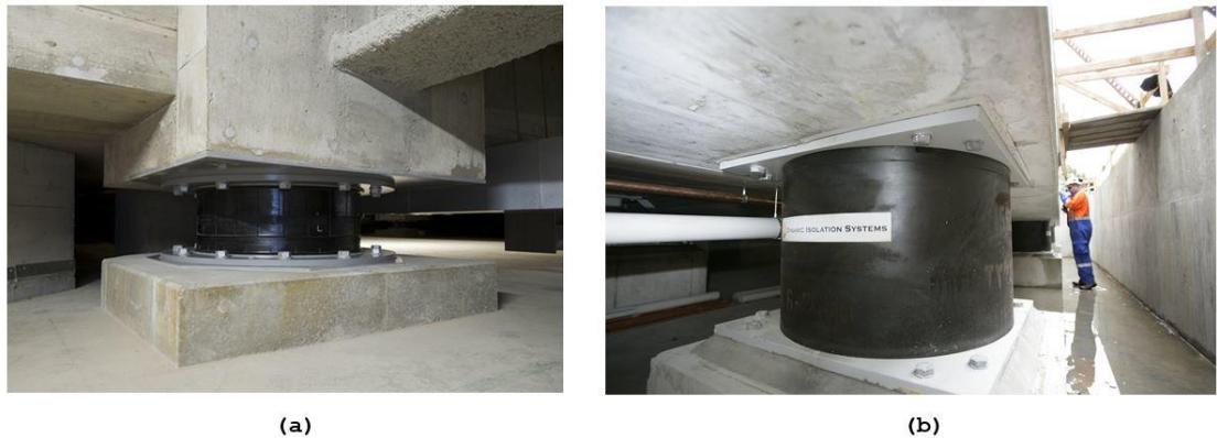
Fig. 1. 4 Elastomeric isolators applied at the ground level of earthquake-resistant buildings, source: www.ibec.or.jp/jsbd/AR/tech.htm .
