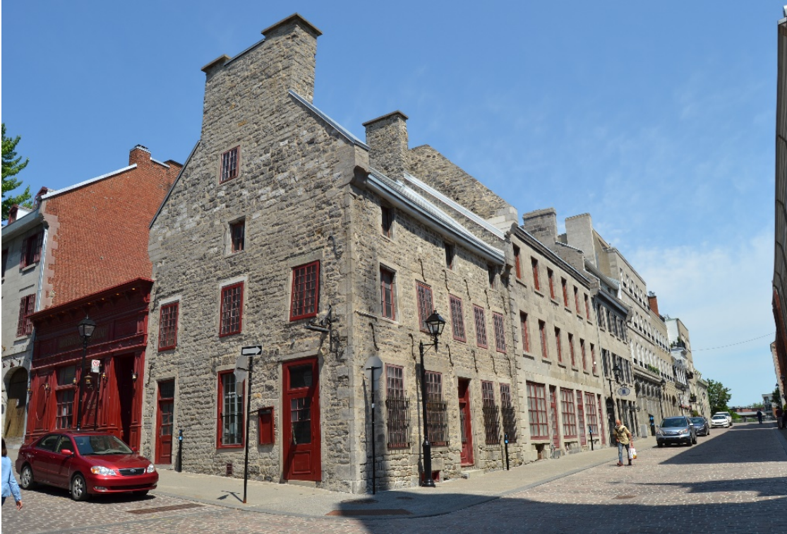
Figure 7- 20 Old tie rods at the level of the slabs in both sides of this old house in the Old Montréal.
