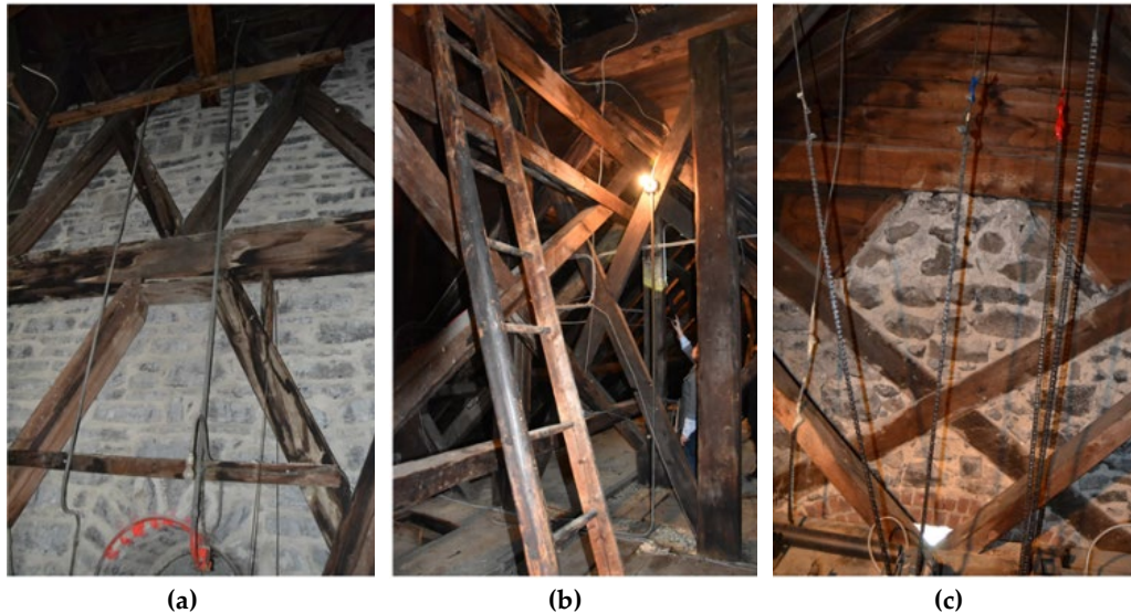
Figure 7- 25 Examples of the structure of the bell tower at the level of connection with the façade: a. the timber structure of the bell tower is adjacent to the façade masonry wall; b. the structure of the roof intersects with that of the bell tower; c. the timber structure of the bell tower starts inside the masonry of the façade ('pan de bois').
