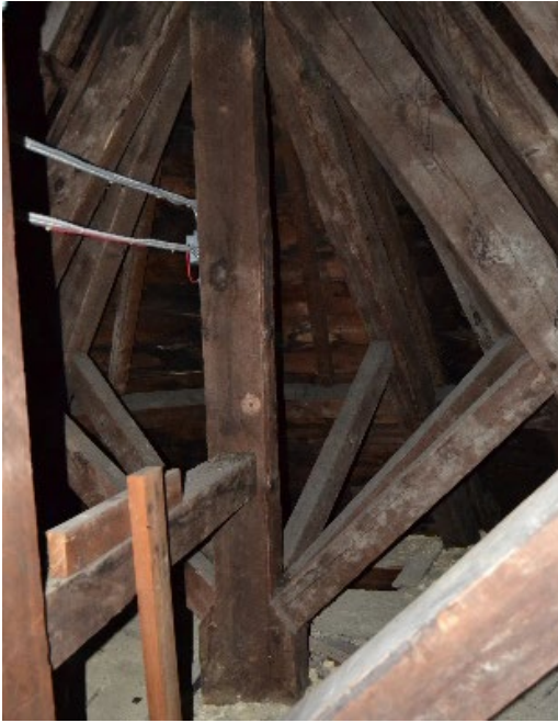
Figure 7- 44 Radial structure of the apse.
