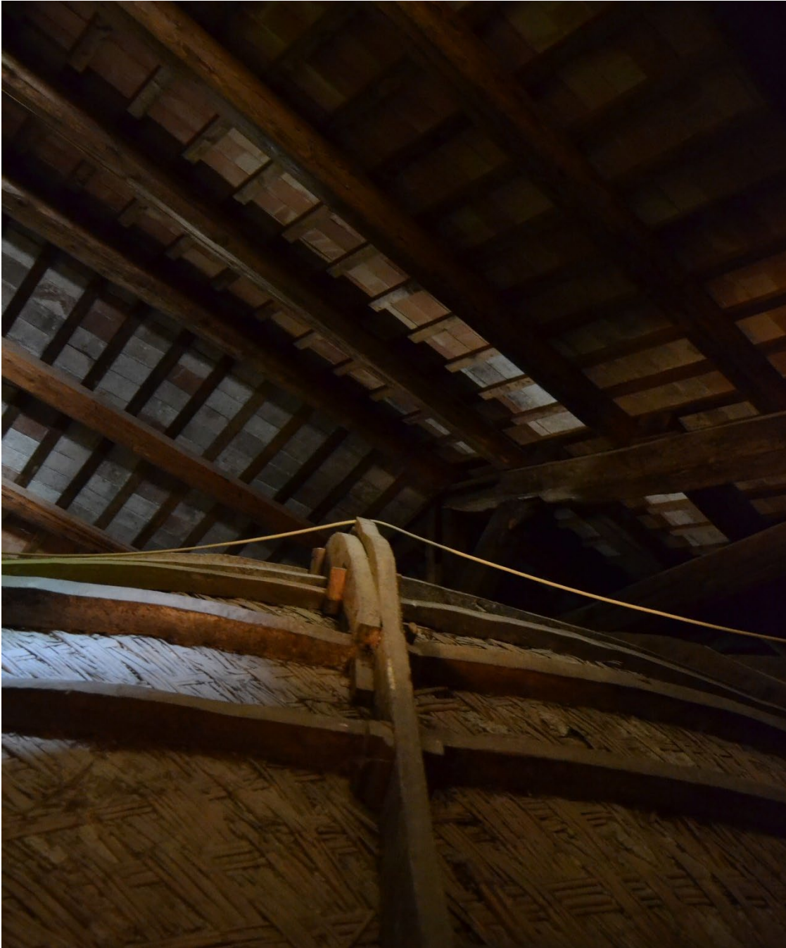
Figure 3- 5 Types of vaults found in the visited churches: a. vault made of bricks laid vertically; b. vault realized with the bricks laid horizontally; c. reed vault with the detail of the connection with the walls; d. reed vault with the detail of the supporting timber structure.
