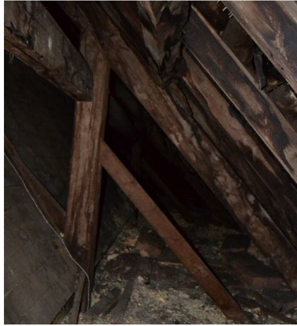
Figure 7- 45 Pillar from the nave, connected with the correspondent truss.
