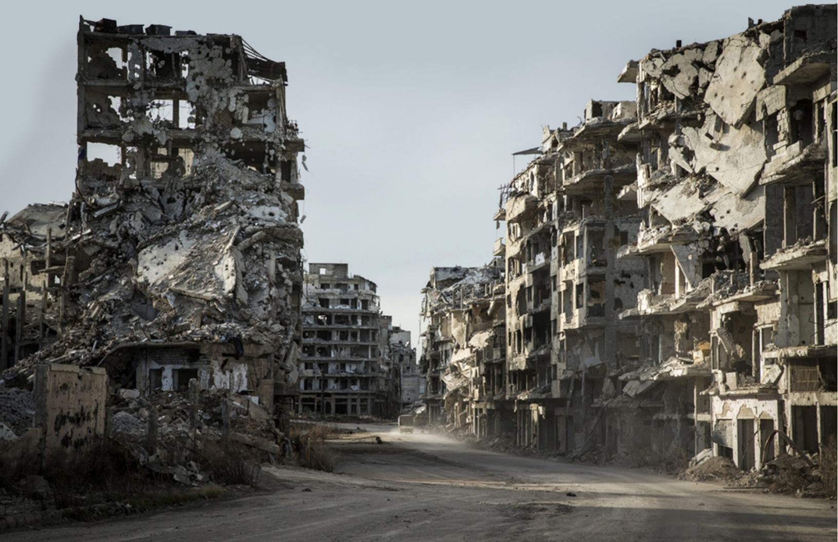
FIGURE 2-6 THE DESTROYED NEIGHBORHOOD OF KHALIDIYA IN THE OLD CITY OF HOMS, SYRIA (UNHCR/ANDREW MCCONNELL)
