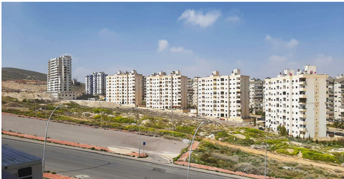
FIGURE 6-16 THE HOUSING UNITS FROM DUMMAR (BY THE AUTHOR)
