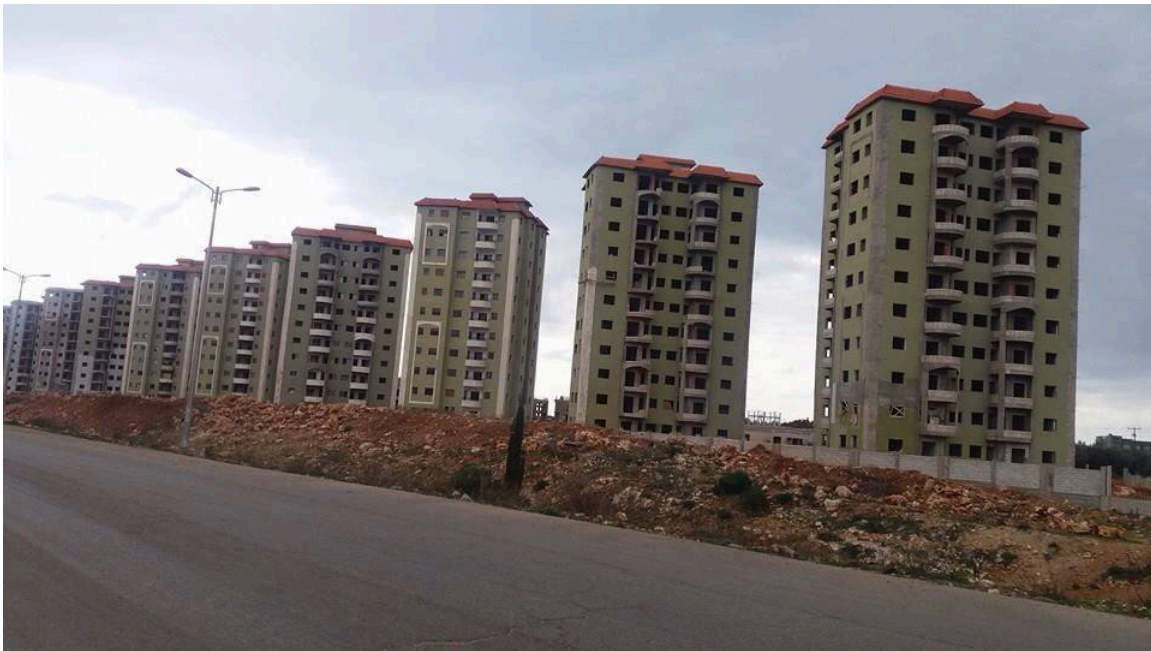
FIGURE 4-9 AL-BASEL SUBURB – FIRST PART OF THE YOUTH RESIDENTIAL PROJECT IN TARTOUS (SOURCE: © ALWATANONLINE.COM)
