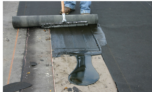
Figure 1.7: Application of a roofing adhesive
