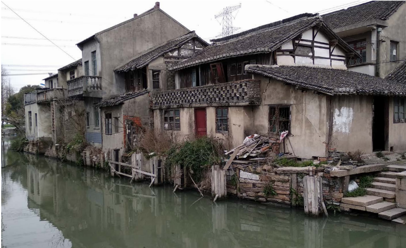
Figure 37. Empty houses waiting to be demolished
