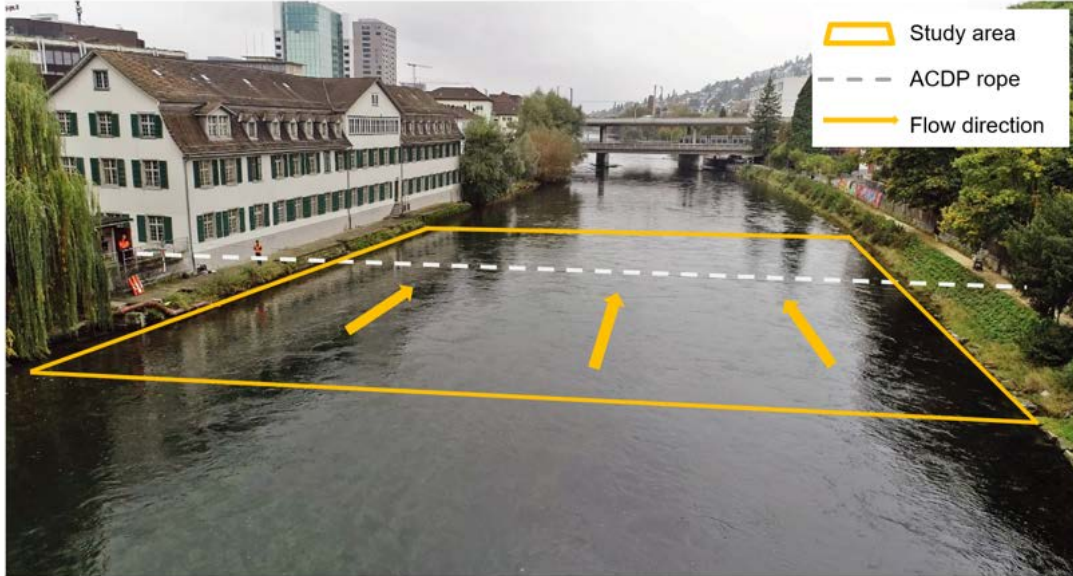
Figure 3.1: Photo of the Limmat - Zürich Unterhard gauging station. On the image are marked: the flow direction (arrows); the area within which the surface velocity is computed through AIV (sold line); the rope used to control monitoring instruments such as the ACDP (dashed line).
