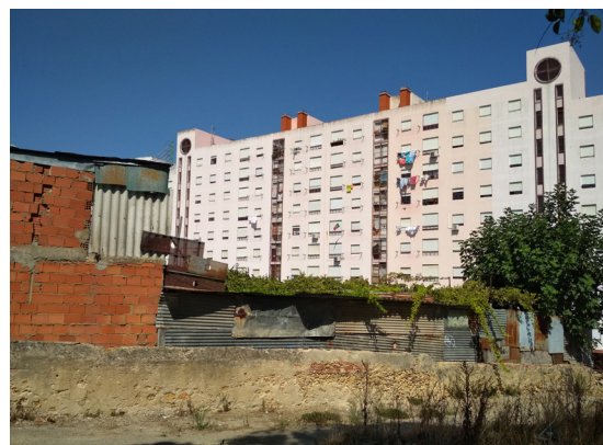
Photo 48: View of social housing in the area of Marvila
