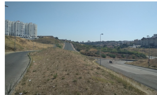
Photo 53: View of urban context south of intervention site
