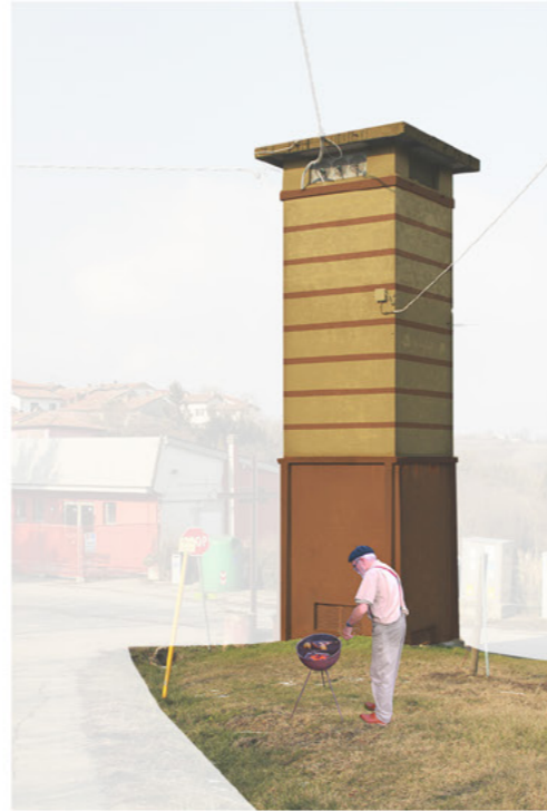
ENEL TOWER Two-tones painting
