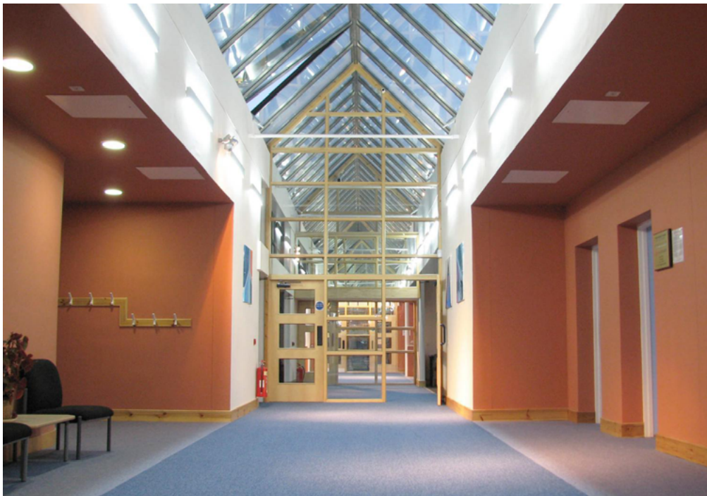
Figure 4.17 'Gull wing' roof for natural light
