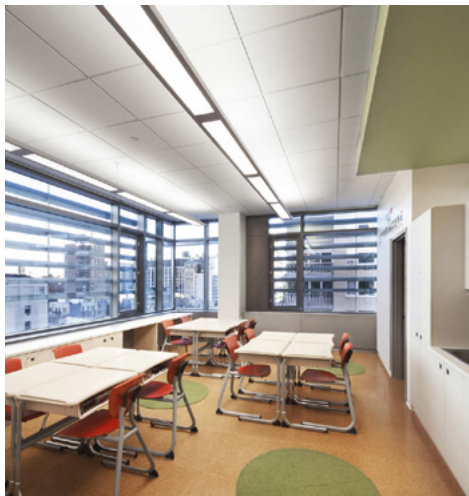
Figure 4.30 Windows with aluminum sunshades
