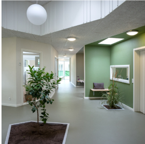
Figure 4.44 Special acoustic panels used in the ceiling
