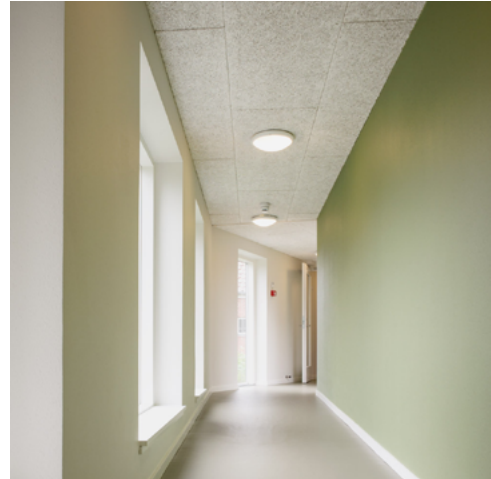
Figure 4.45 Special acoustic panels used in the ceiling
