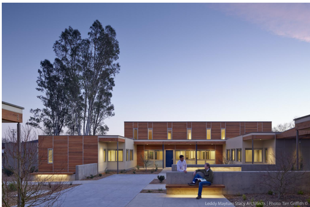
Figure 4.36 The outside view of Sweetwater Spectrum Community (Source: https://www.archdaily.com/ )
