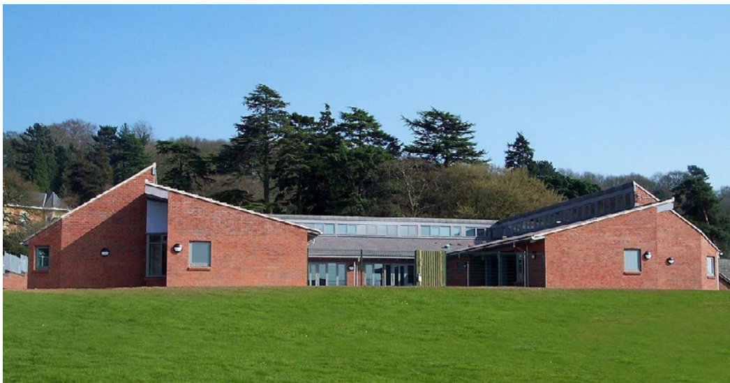
Figure 4.2 Overview of Sunfield Residential Unit (Source: Ga Architects)
