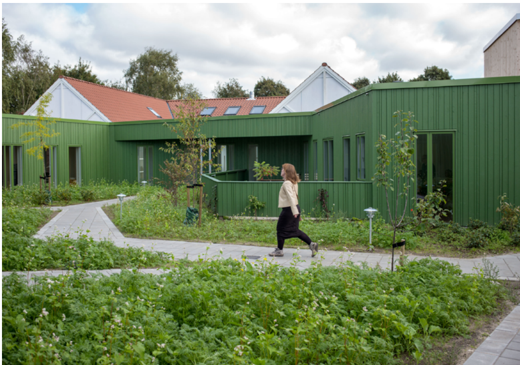
Figure 4.39 Outside view of the senior house (Source:www.troldtekt.com)
