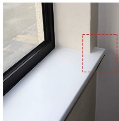
Corner of windowsill
