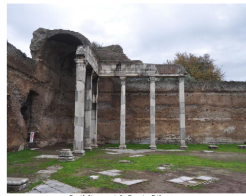
Building with Doric Pilasters (Current English Language Guide Book (B. Ademברי) or E. Salza Prina Ricotti .)
