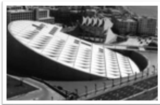
Figure 28 The inclined roof which forms a challenge for maintenance processes Head of Preventive Maintenance Management Department(2010)-Open Interview, Bibliotequa Alexandrina – Alexandria, July 2010
