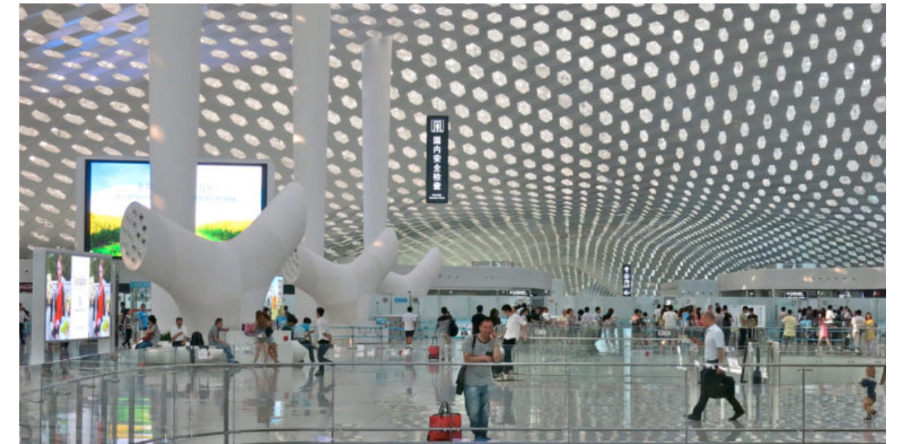
Figure 78. The Shenzhen Airport, by Massimiliano Fuksas, has a wave-like skin that was parametrically designed by a single person, using scripts that took into account necessary structural and daylighting requirements. Source: https://d1xchyou513y0i.cloudfront.net/wp-content/uploads/2017/10/2017442111-Shenzhen-Airport-768x511.jpg
