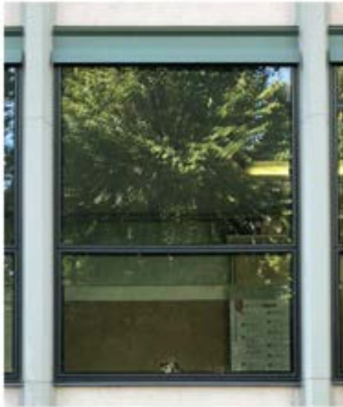
Typical window in east elevation
