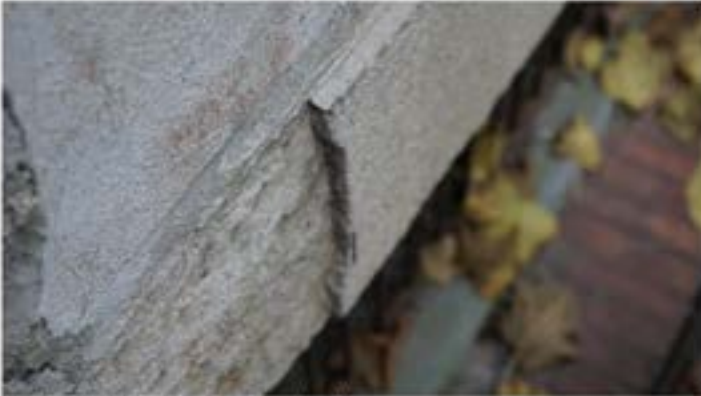
Finishing detached partly (photo from the side)
