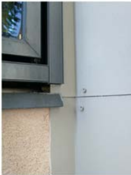
Detail of a window in east elevation
