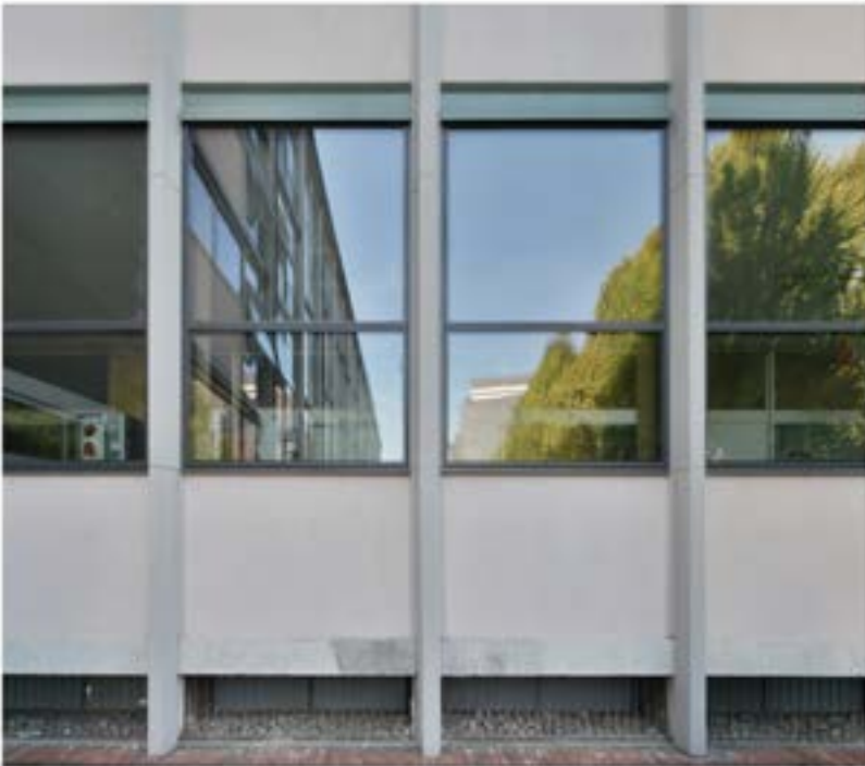
view of east facade
