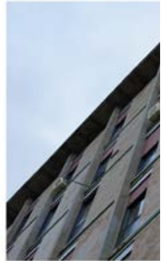
▲ Façade of convitto
