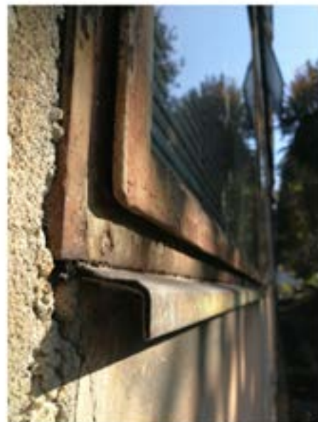
Detail of a window in west elevation
