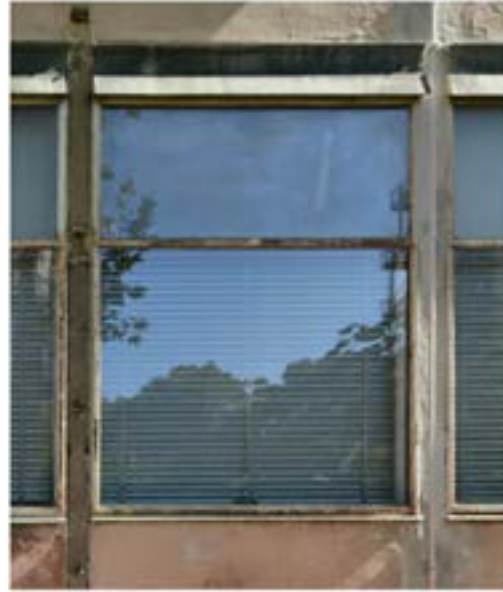
Typical window in west elevation
