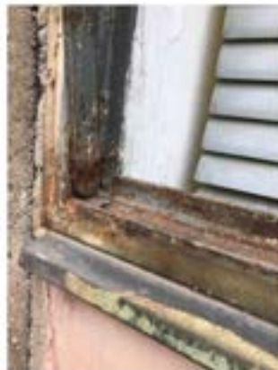
corner of the frame
