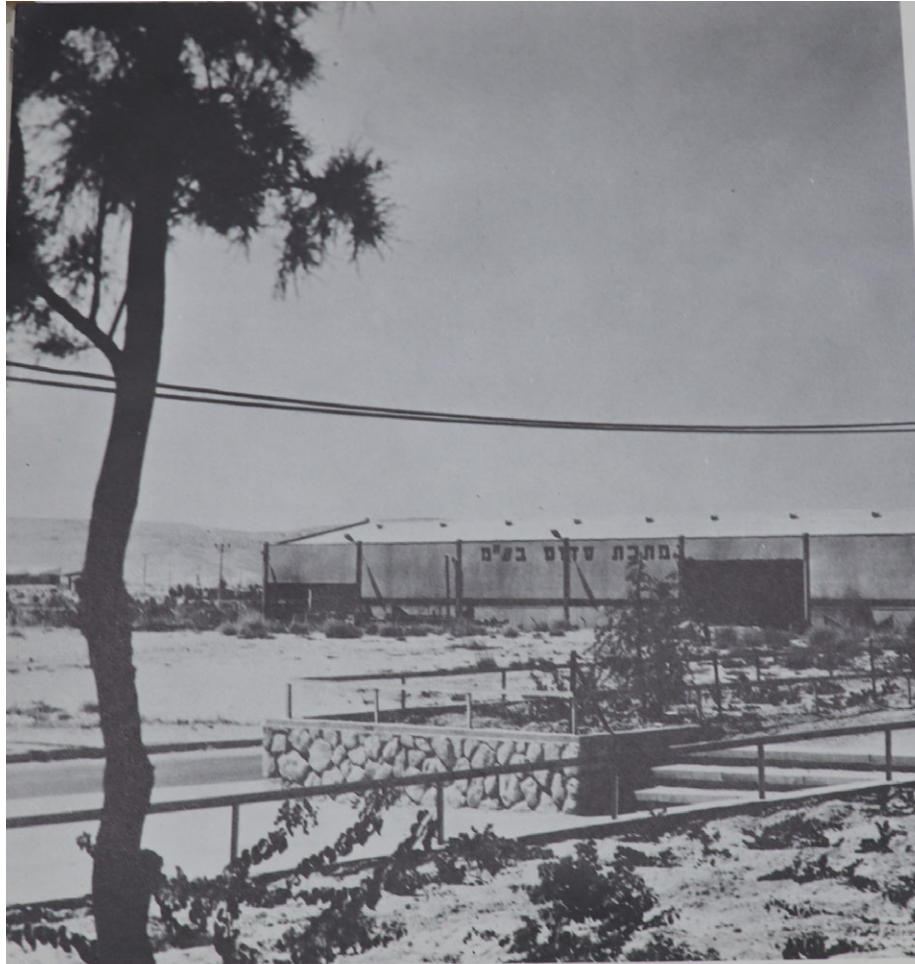
Figure 92-93: The sakum Sdom factory . In: Municipality of Dimona, Dimona – story of a city , Ahdot press, Tel Aviv, 1973.p. 11-12
