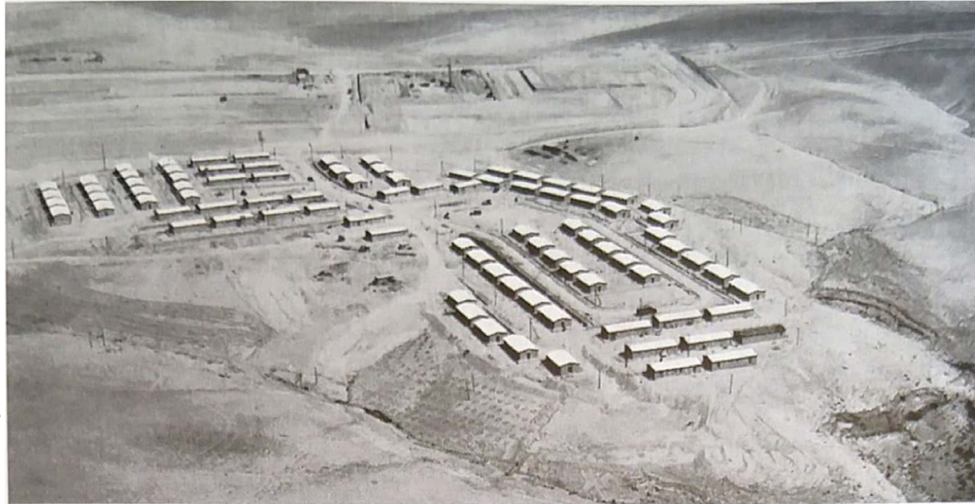
Figure 36: Aerial view of the transition camp of Arad (1963) in Z. Efrat, M.Yagid-Haimovich, The Israeli project – construction and architecture 1948-1973 , Vol.2, Tel Aviv Museum for art, Tel Aviv, 2004 p.787
