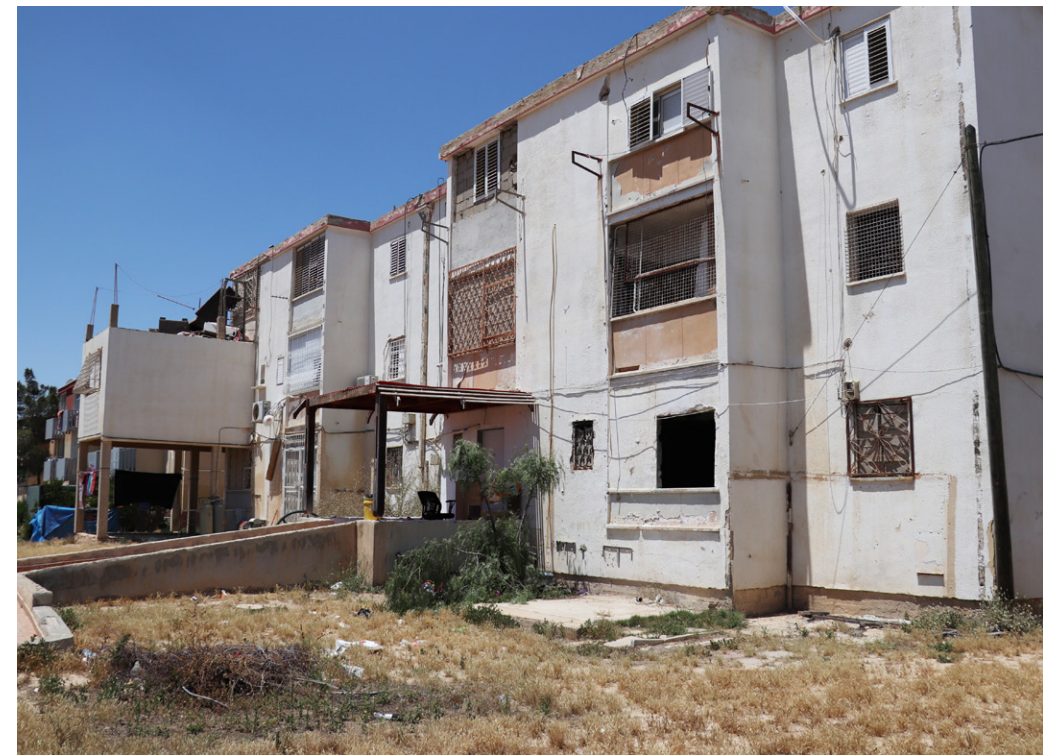
Figure 144-145: Abandoned structure in Baba-Sali street 04.2020
