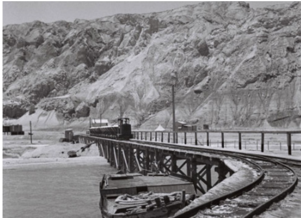
Figure 62-63: The worker's camp in Sdom . In: Xnet online architectural magazine 20.3.2020
