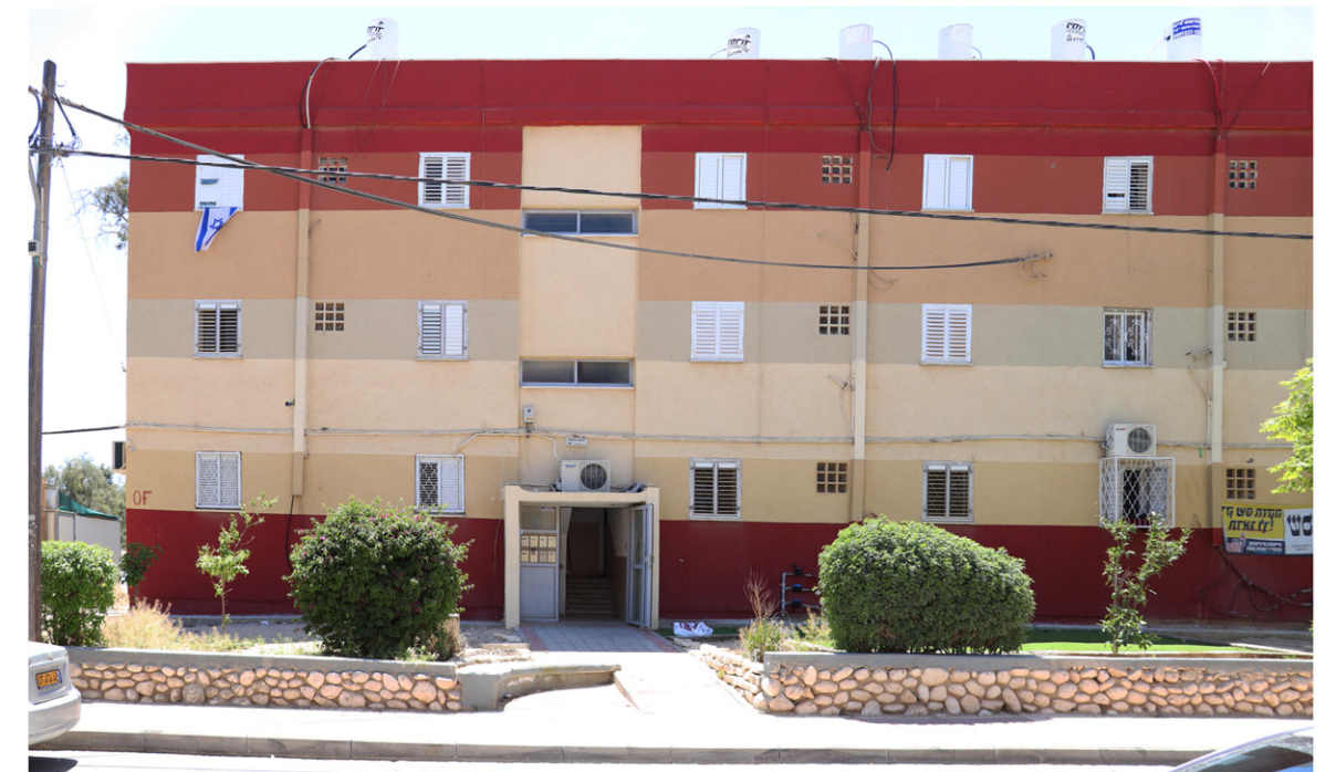
Figure 189-190: Main facade of un-restored and restored of the 139 model 04.2020
