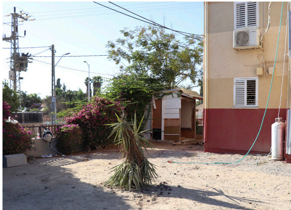
Figure 171-172: illegal construction in the Shivat Ha Minim neighborhood. 08.2019
