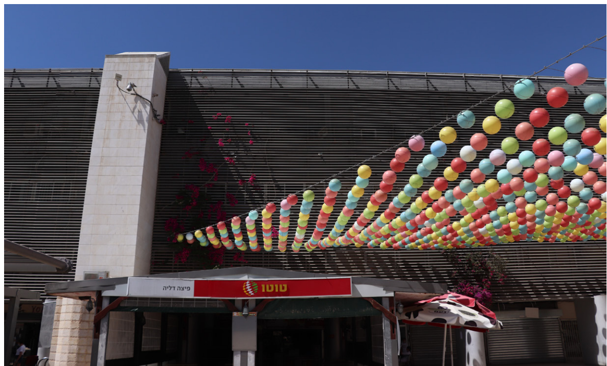
Figure 236: The southern facade of the municipality's building 04.2020
