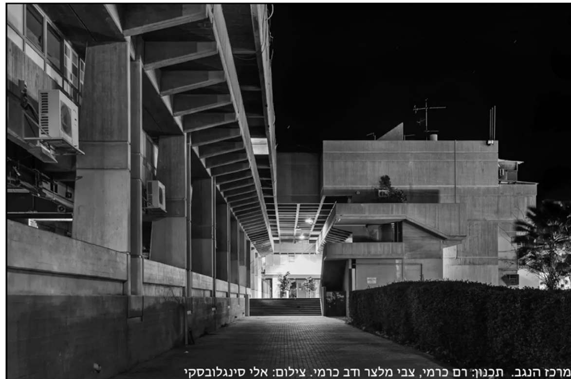
Figure 27: The Negev Center planned originally by Ram Karmi and Zvi melzer (1959). In: E.Singalovski, 'Sunburn exhibition' the Association for promoting of Brutalist Heritage in Israel website.
