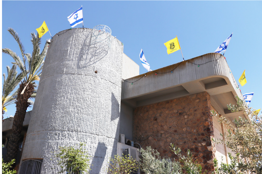
Figure 265: Exposed concrete and the original local stone cladding 04.2020
