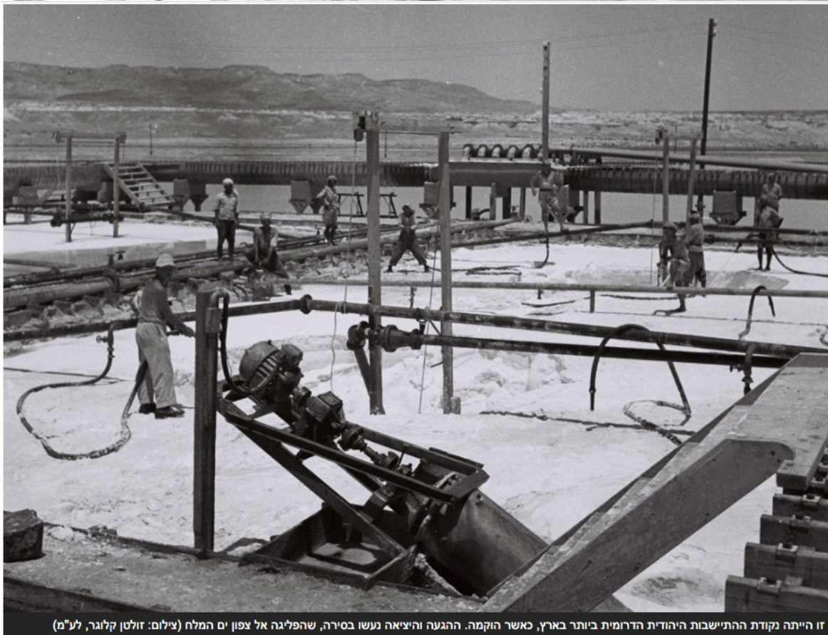
Figure 60-61: The worker's camp in Sdom . In: Xnet online architectural magazine 20.3.2020
