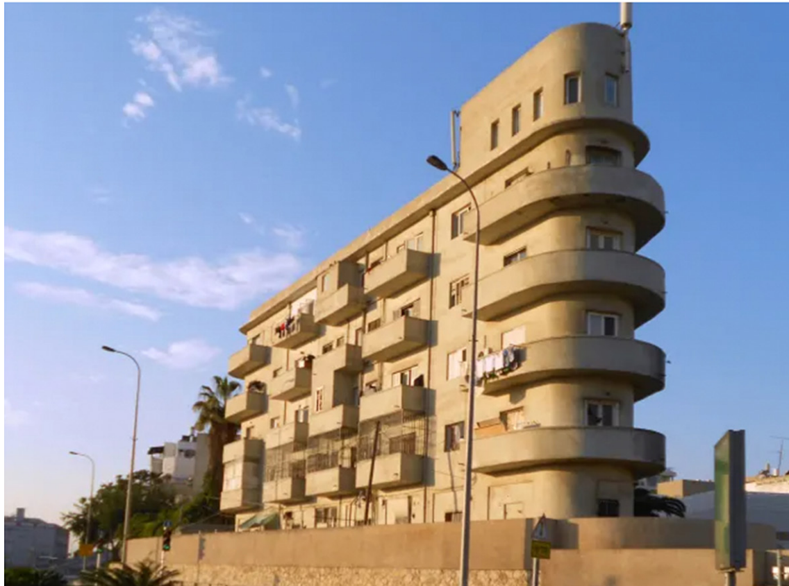
Figure 25: The ship house planned originally by Shimon Hamdi Levi (1934-1935). In: The official Bauhaus center in Israel website.
