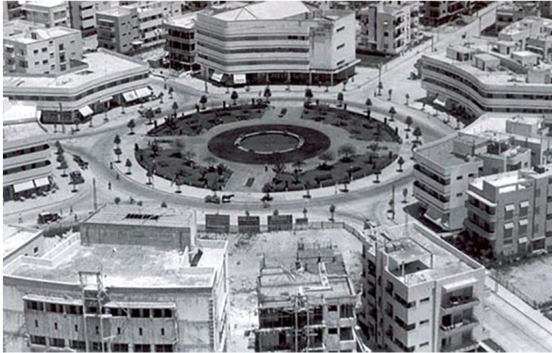
Figure 24: Zina Dizingoff square planned originally by Genia Averbuch (1938). In: The official website of the Municipality of Tel Aviv- Juffa.
