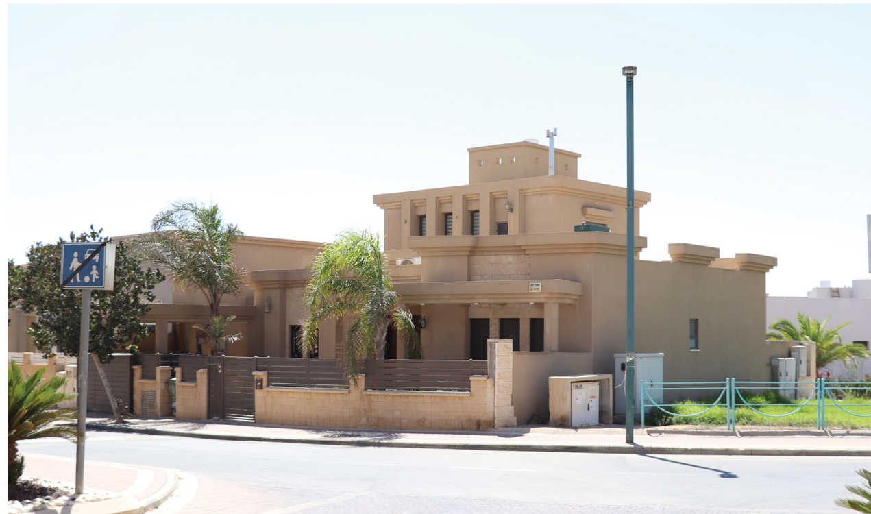
Figure 124-125: Structures From Benei Bitha in Dimona . 08.2019
