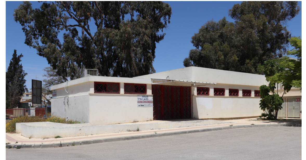
Figure 215: The Dining structure of the Yoseftal school - Southern facade 04.2020
