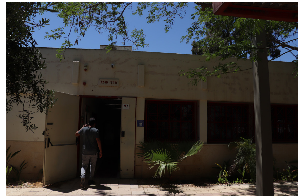
Figure 216: The Dining structure of the Yoseftal school - Eastern facade (It is still possible to see the sign indicates of the function) 04.2020
