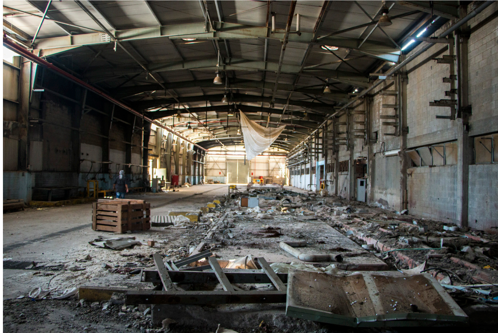
Figure 126: Abandoned manufacturing hall at Kifan Dimona 08.2019
