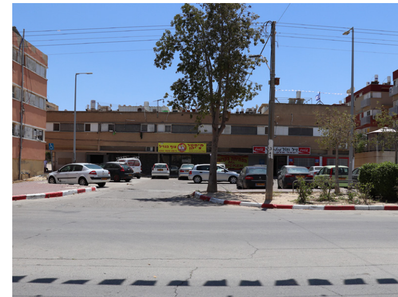
Figure 208: The commercial center structures inside the 'Best' Neighborhood 04.2020
