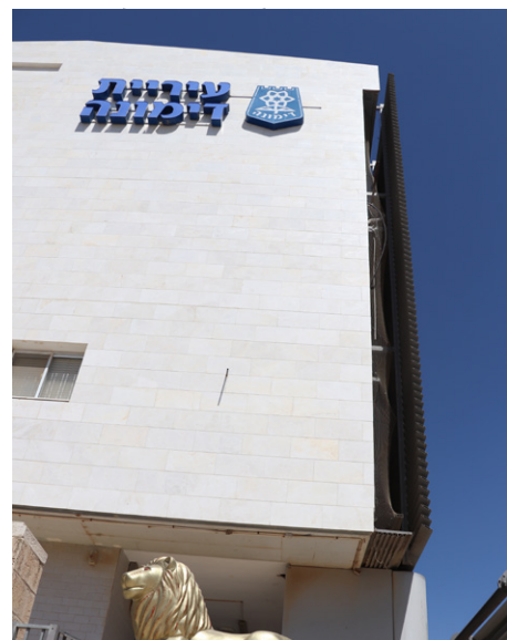
Figure 235: The western facade and a section view of the recent adjustment 04.2020
