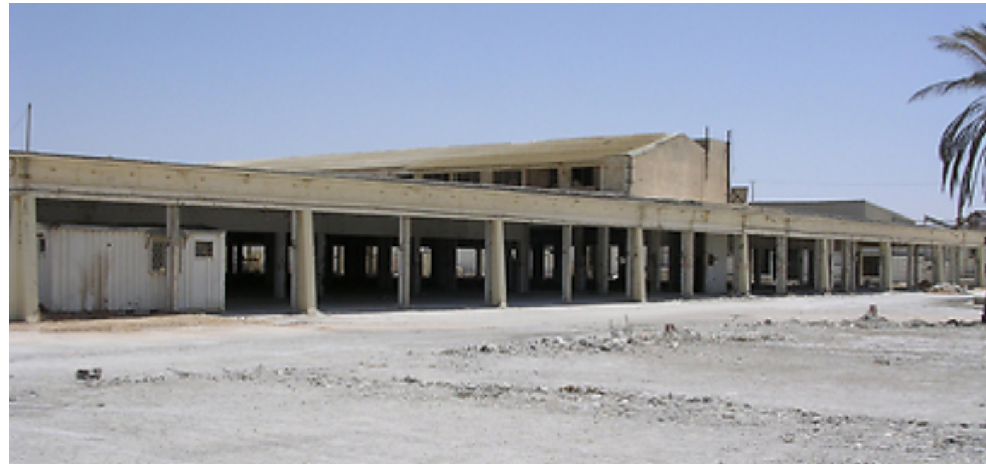
Figure 167: The Abandoned structure of the 'Dimona textile' factory in the southern industrial district. In: H.Zi'on , The factory that wanted to be a mall , "Yediot Ahronot" daily newspaper, 10.03.2012.
