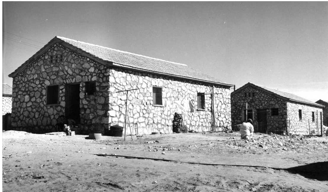
Figure 79-80: The construction of the Blockon type in Dimona. Unknown photographer, Unknown year. In: The Tuvyah archive of the Ben Gurion university library, Photo No. 706.81.F2.99.D1, 706.81.F2.99.D4
