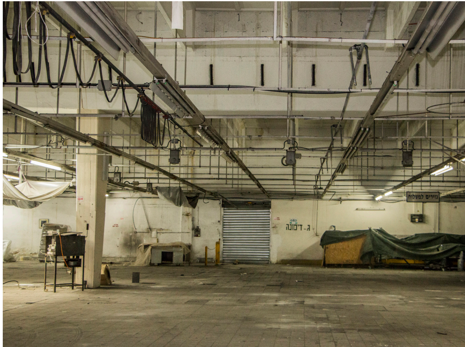
Figure127: Abandoned sewing department at Kittan Dimona. 08.2018
