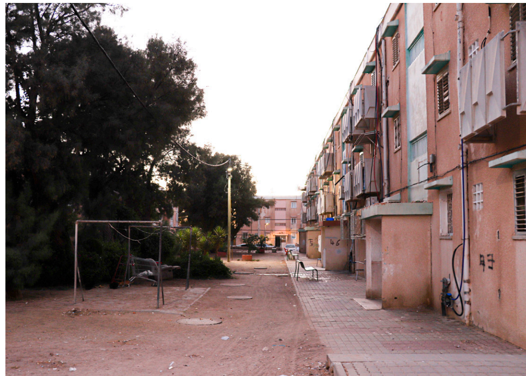
Figure 174 : Low quality of the public space in Yosheftal neighborhood. 08.2019
