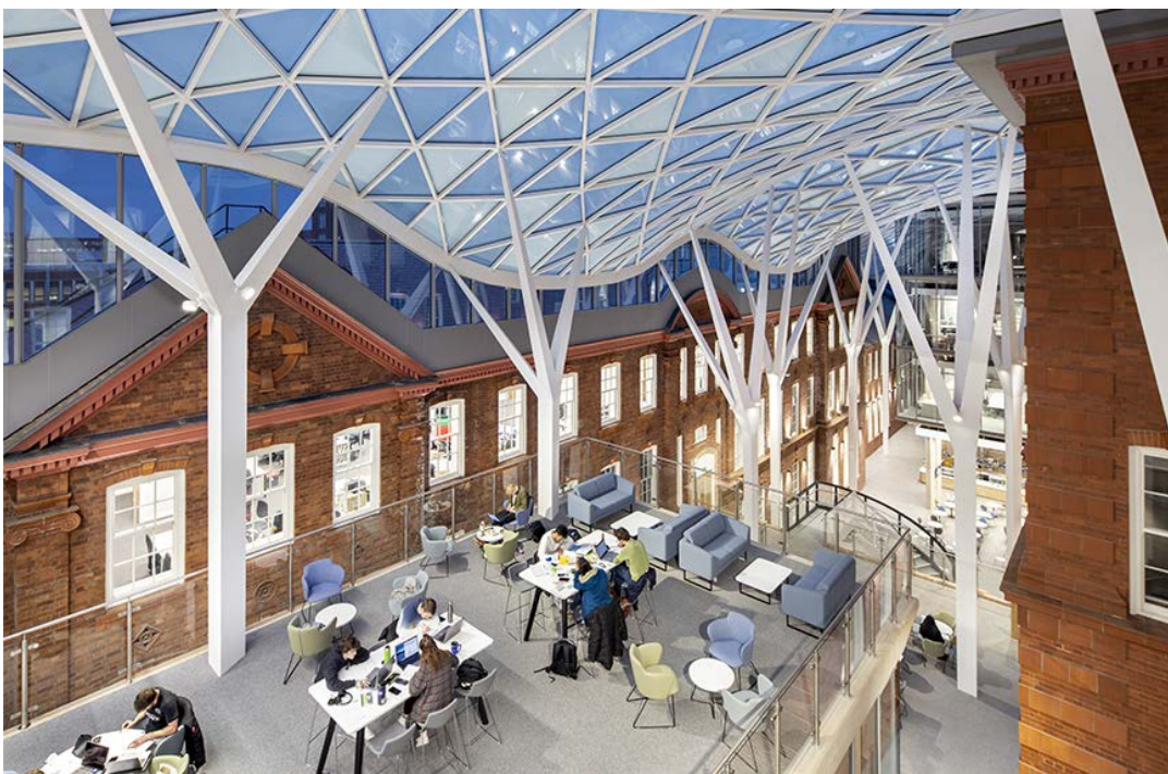
Image 26. The project exemplifies a successful initiative of re-discovery and refurbishment of overlooked possibilities on campus. (The University of Sheffield, 2020)
